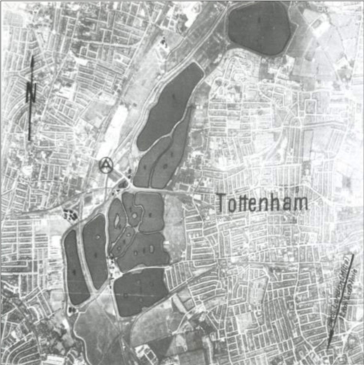
London- Tottenham Water treatment works and reservoir TN 81
