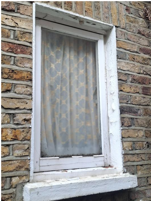
Rear Side Ground Floor Window
