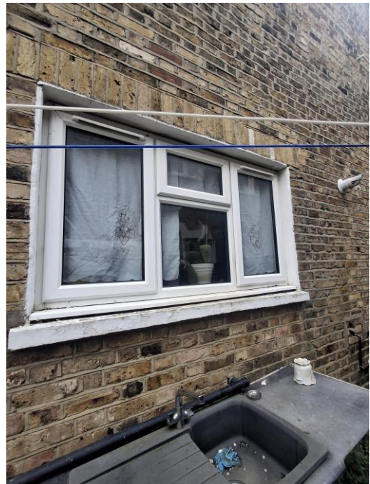
Rear Side Ground Floor Window
