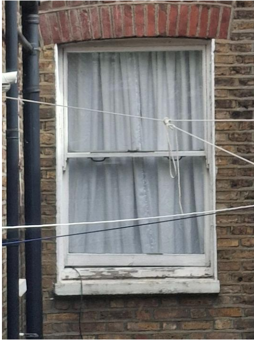
Rear Ground Floor Window
