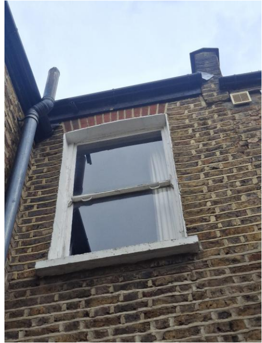
Rear First Floor Window
