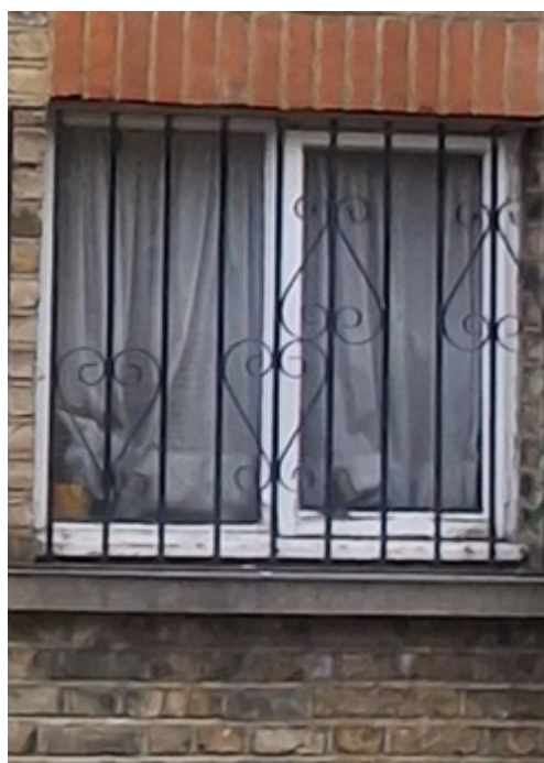
Rear End Ground Floor Window
