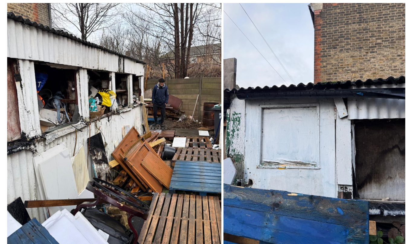
Figure 2 – Existing Site Photographs
