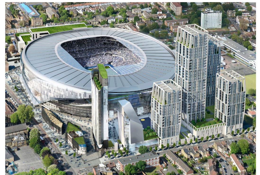
FIGURE 72. Aerial View of the Stadium Southern Development
