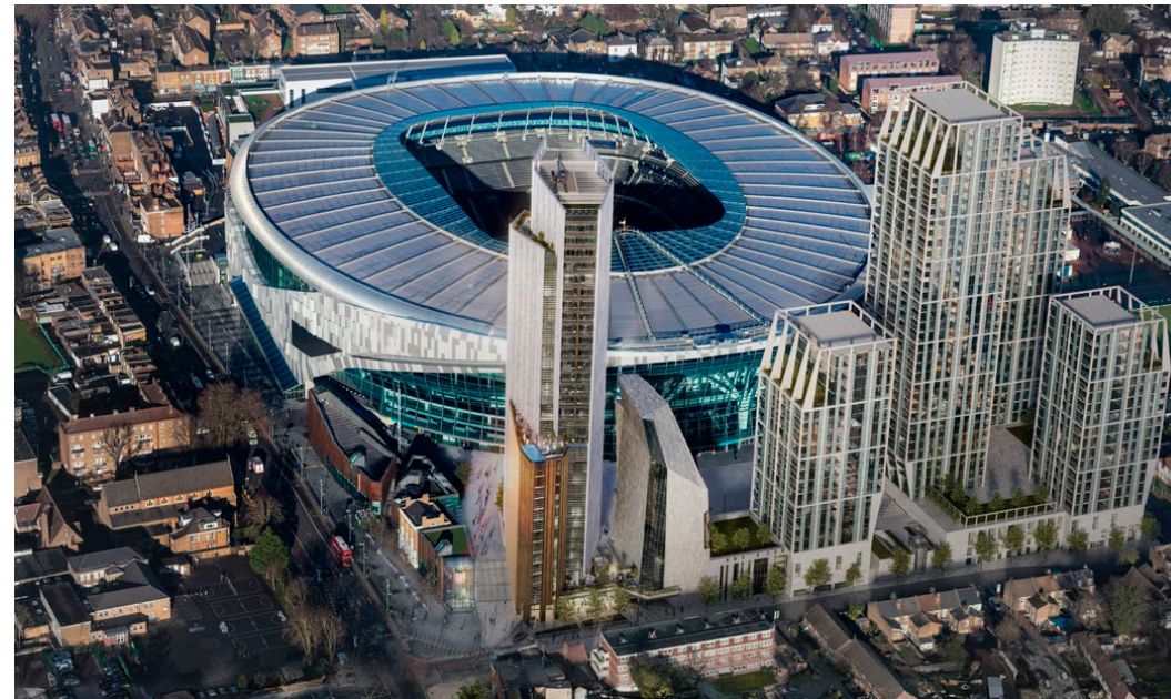
FIGURE 73. Southern Development Aerial Overview
