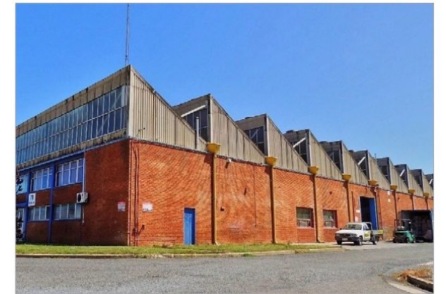
FIGURE 85. Heritage (Sawtooth Factory Roof)
