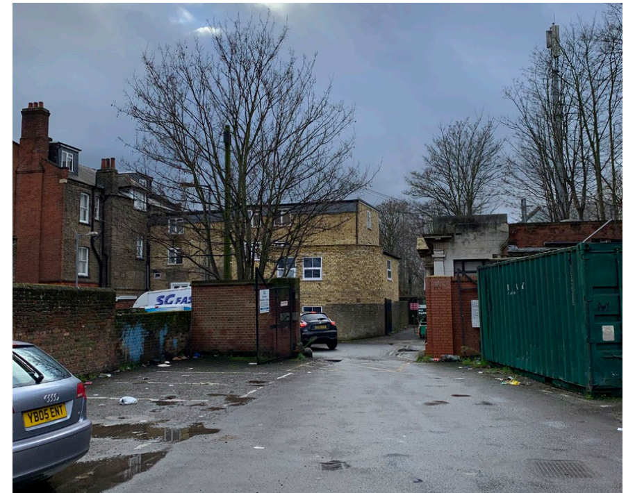
FIGURE 187. Commercial Car Park Accessed Through 551 Alleyway
