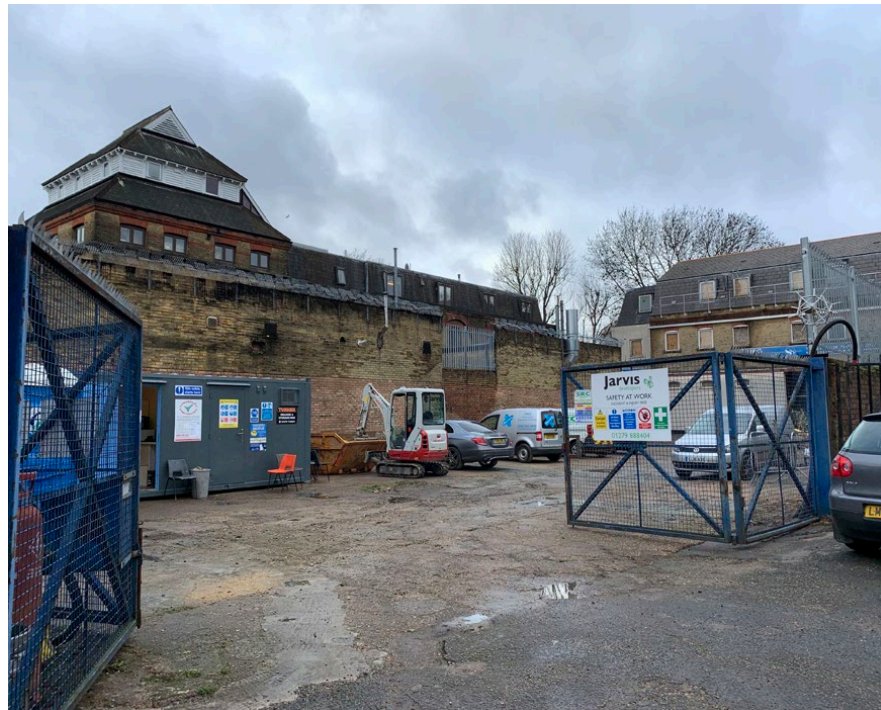
FIGURE 183. Developer's Yard Accessed Through 577 Alleyway
