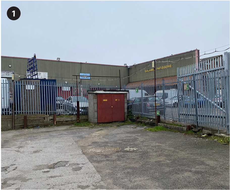
FIGURE 53. North West Corner Along Brunswick Square
