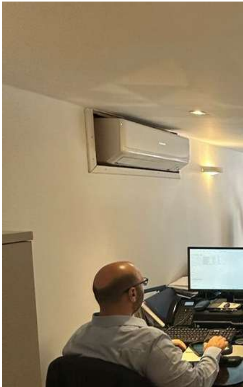
Existing image showing the air conditioning unit hung off the brick wall with the plasterboard cut around.
