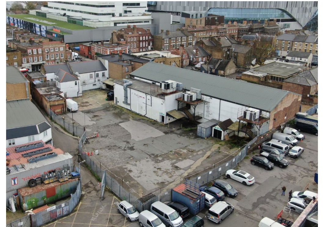
FIGURE 7. The Printworks looking south east (2)
