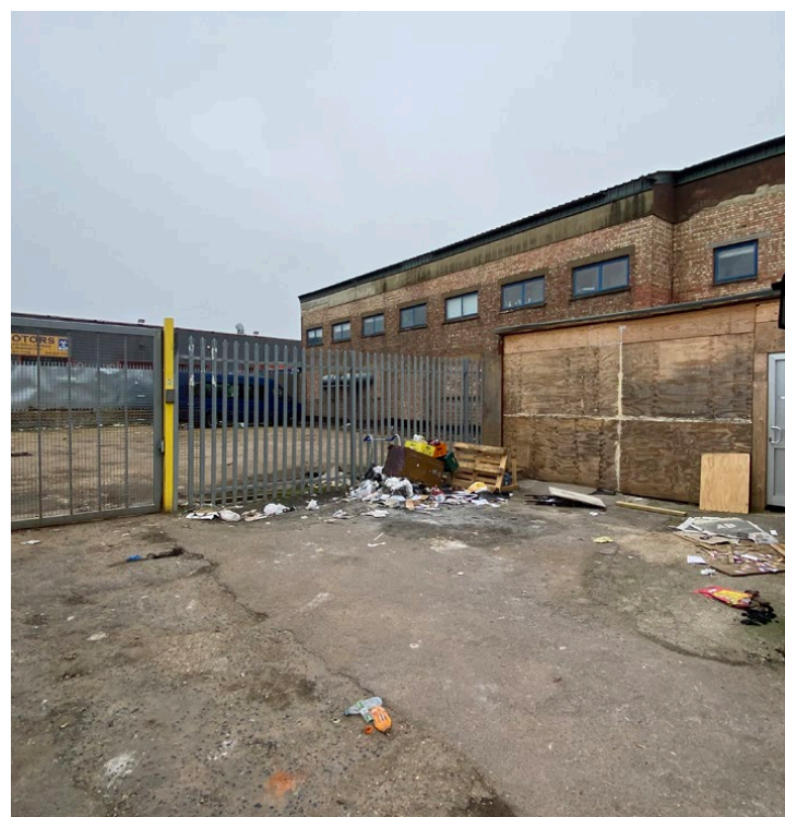
FIGURE 15. Small car park in the south west corner. (3)
