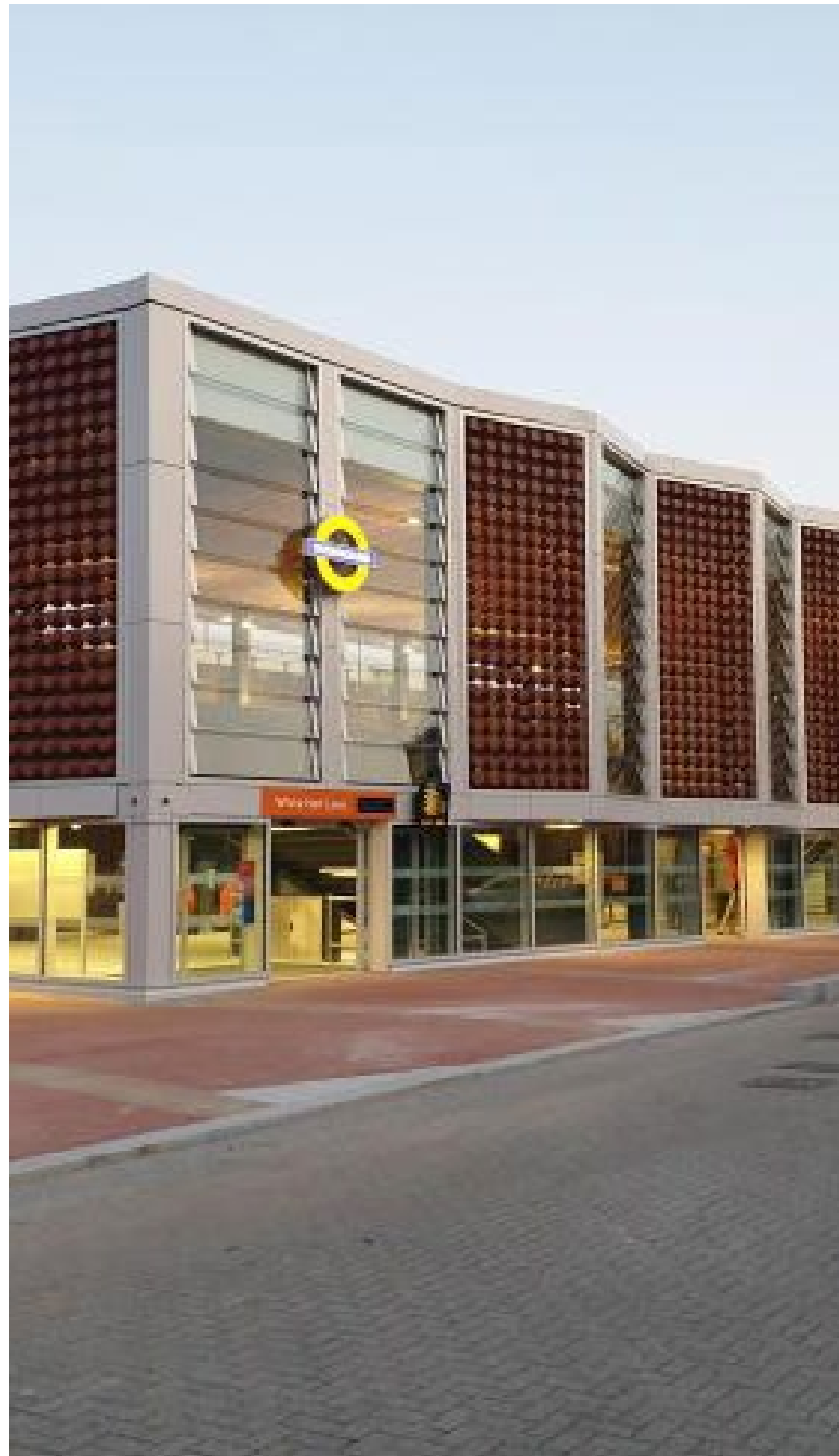
FIGURE 21. Newly Refurbished White Hart Lane Station
