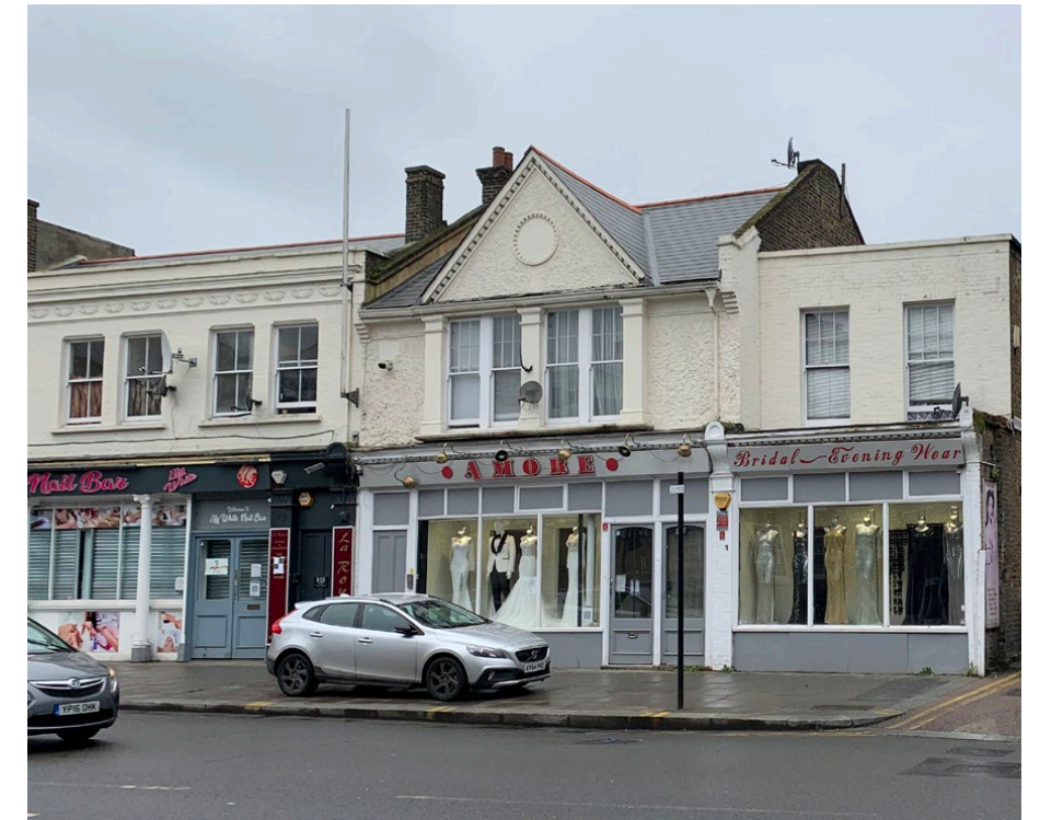
FIGURE 11. Nos. 823-829 High Road (2)
