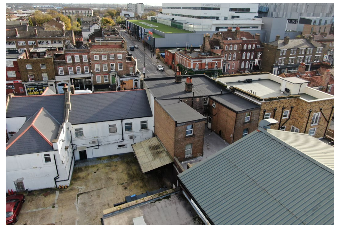
FIGURE 16. Rear of nos. 819-827 High Road (4)
