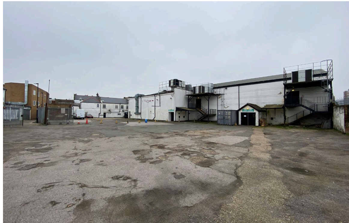
FIGURE 13. View of large car park in the north west of The Site (1)
