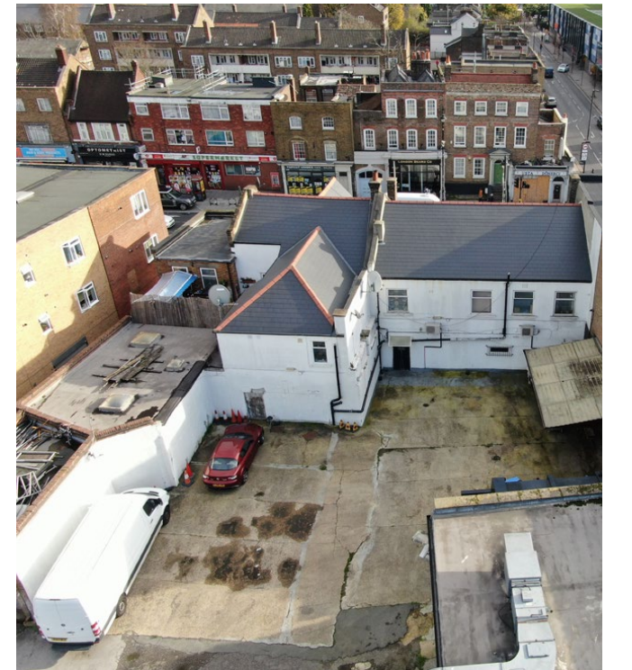
FIGURE 14. Rear of nos. 823-829 High Road (2)
