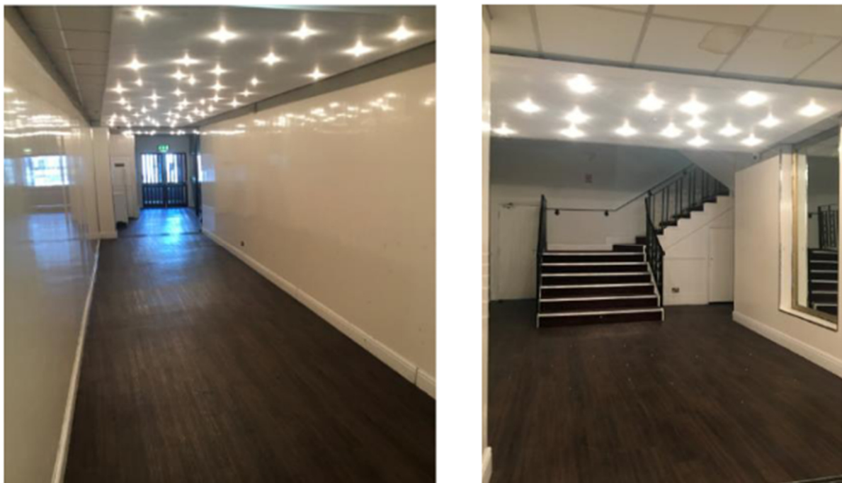
Figure 32 extract showing the late C20 claddings of the ground floor spaces, generally dating from 1993.
