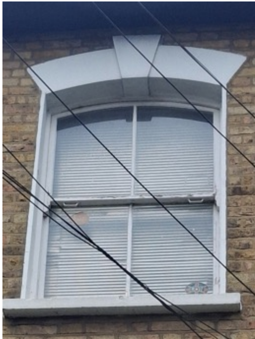
Front Second Floor Window
