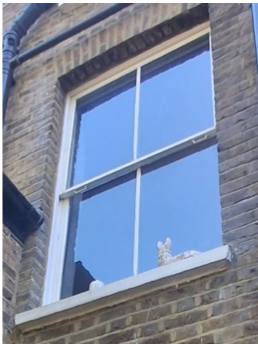
Rear First Floor Window
