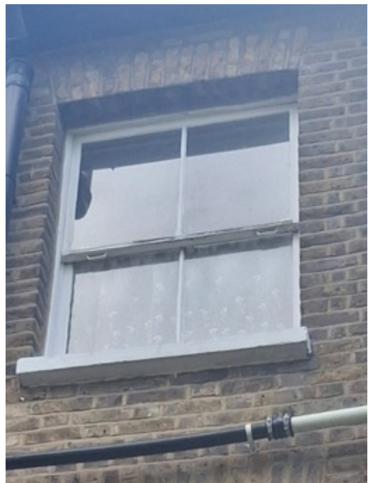
Rear Second Floor Window
