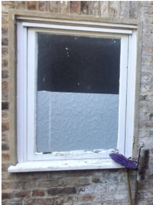
Rear Side Ground Floor Window
