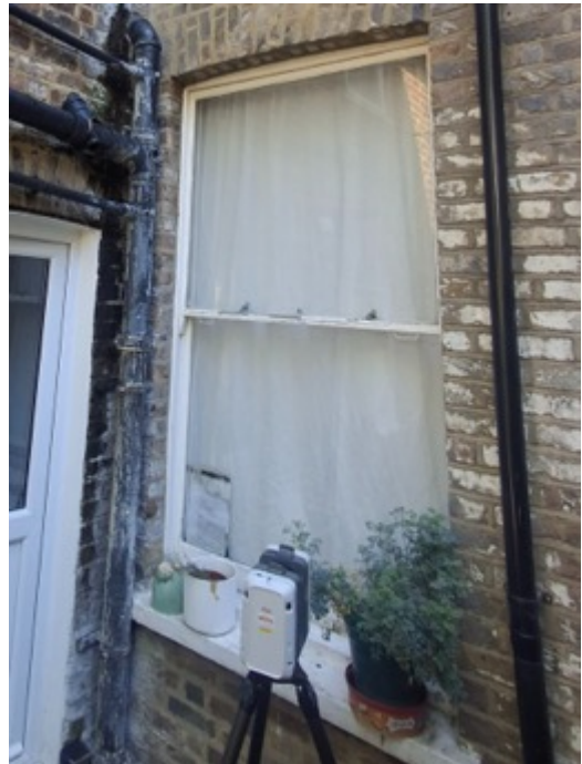
Rear Ground Floor Window
