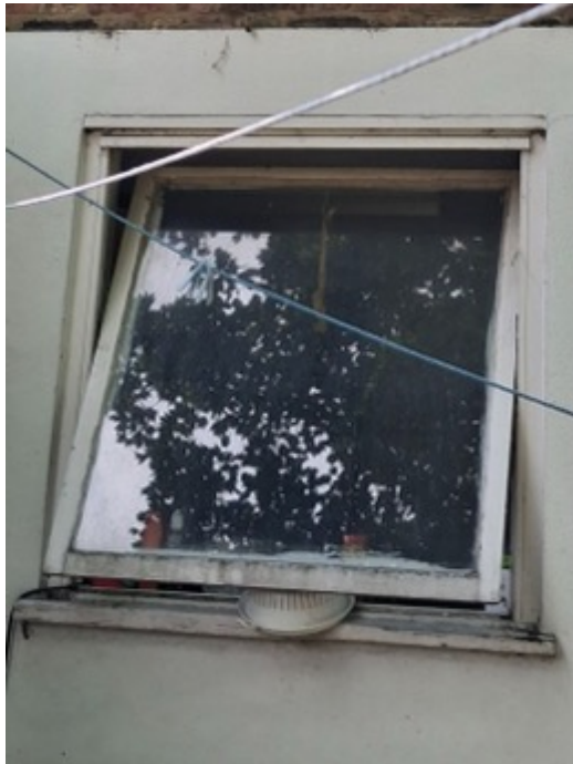
Rear End Ground Floor Window
