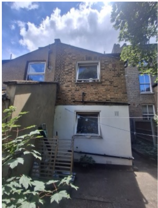
Rear End Elevation (North West)
