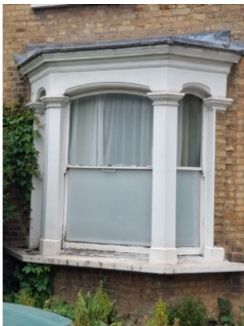
Front Ground Bay Floor Window
