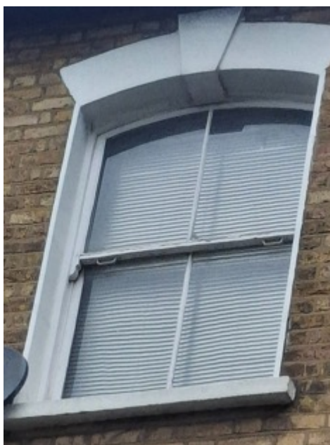
Front Second Floor Window
