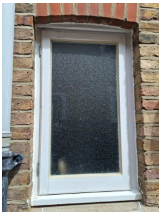
Rear Side Ground Floor Window
