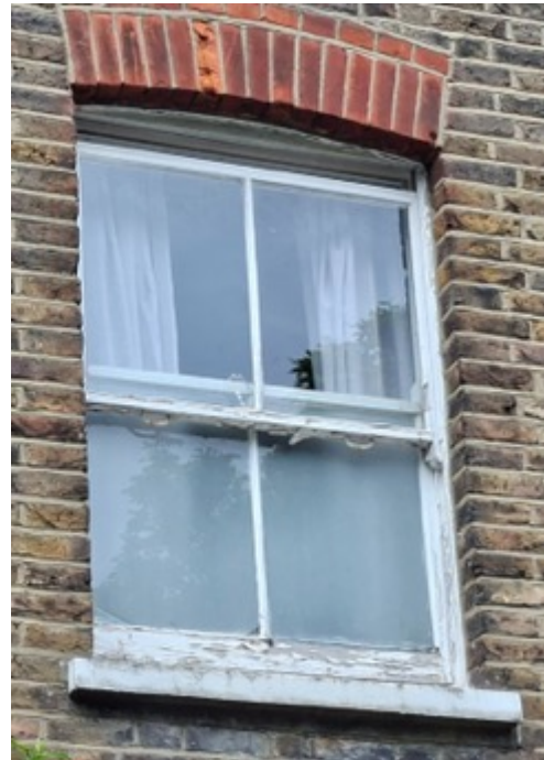
Rear End First Floor Window
