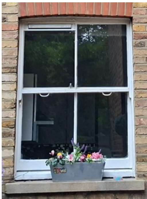
Rear Ground Floor Window
