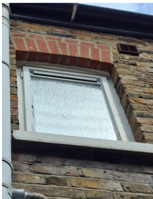
Rear Side First Floor Window
