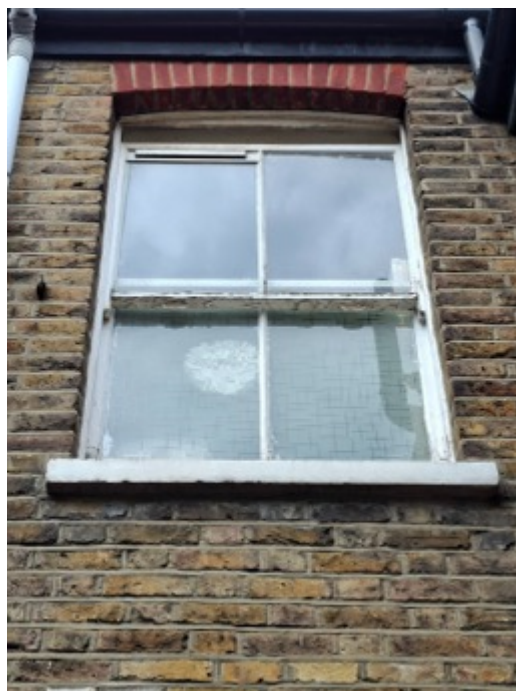
Rear First Floor Window
