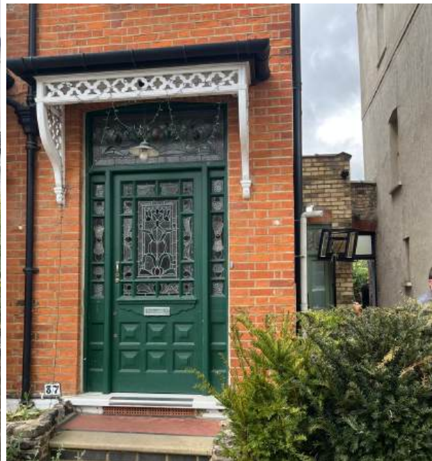
Side gap between Nos.35 and 37
