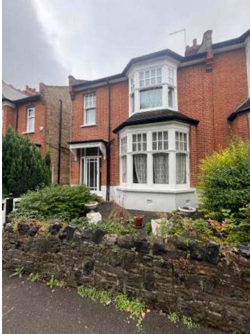
View of 35 Collingwood Avenue from the street
