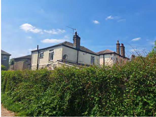
Photo 8 – View of the side/rear elevation (east/northeast)
