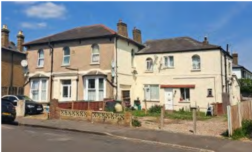
Photo 1 – View of front elevation (south)
