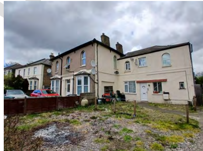
Photo 4: B1 - southwest elevation
