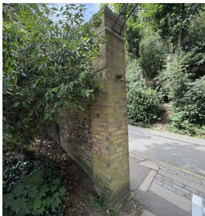
Photograph K- Detail of rebuilt pillar from the opposite side of photograph B as visible from the public realm. There are no blue/grey plinth stones at this location.
