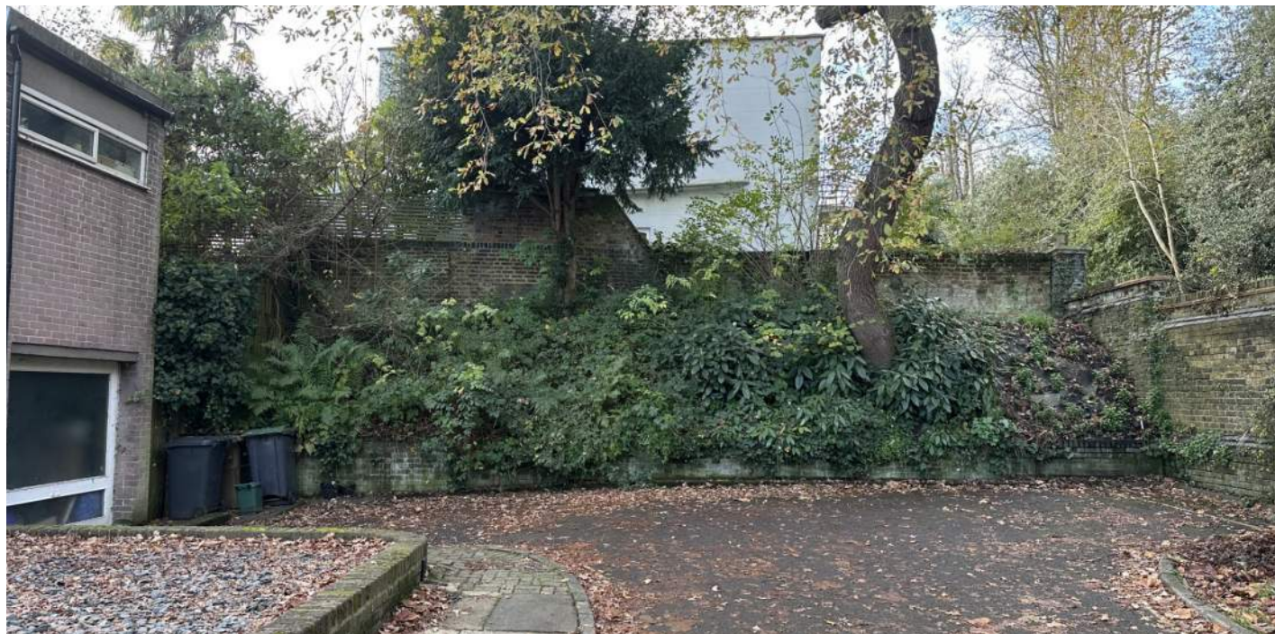
Photograph F - Showing the boundary wall from the Southwood Estate Cul-de-sac road parallel to Southwood Lane. Further photographs below discuss the condition of this wall in greater detail.
