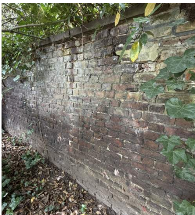
Photograph J - Looking along the length of the boundary wall as hidden behind the bushes with a solid capping stone at the top and simple wall course below.
