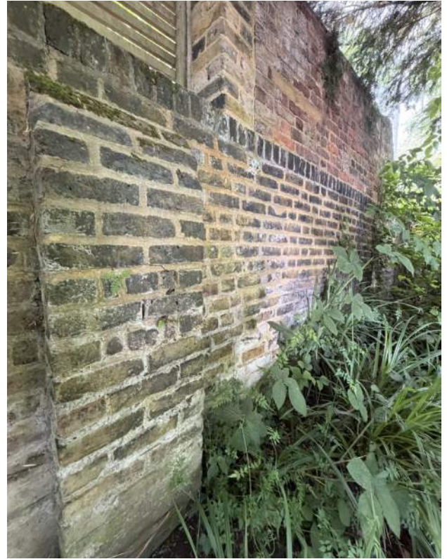
Photograph R - side view (diagonal wall to the left) showing a different buttress style on the boundary wall where brickwork curves up to the top to meet the wall behind it.
