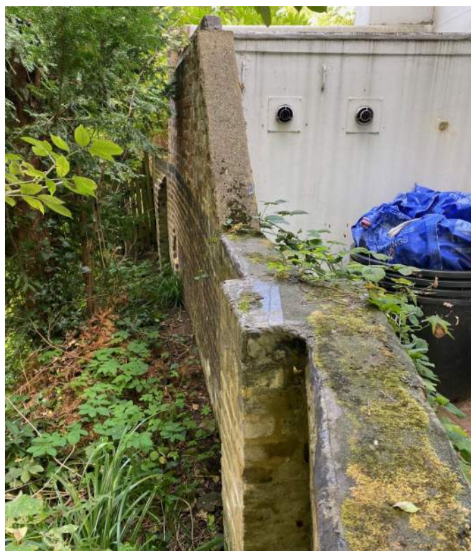
Photograph P - Showing a square topped buttress and the sloping brickwork behind (presumed a later addition)
