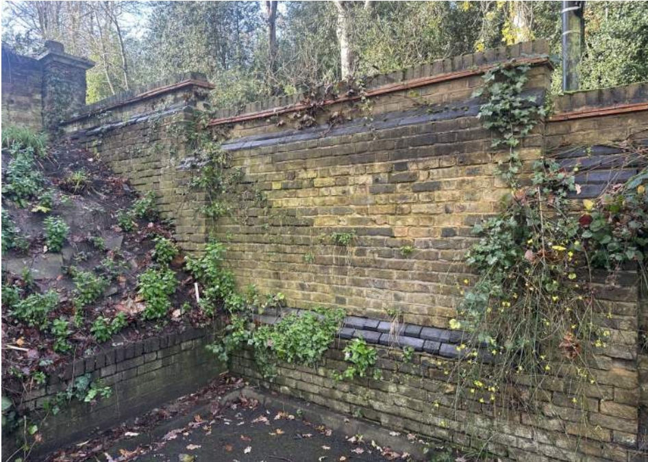
Photograph L (left) - Detailed photograph of the corner of the wall taken during winter. Grey/Blue double course plinth stones are evident at the top of buttresses and where the brick wall thins from a thicker base to a single brick course at the top. Also evident is a header course and double tile detail. The grey linear element at the base of the wall is the the adjoining cul-de-sac road kerb, set forward of and separate from the wall, which is highway infrastructure and not part of the boundary wall. The base of the wall itself carries no plinth or coping stone.
