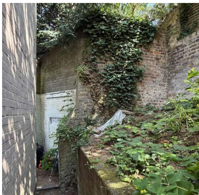
Photograph U - showing the end masonry wall in a predominantly red brick with a chamfered end suggesting the wall was cut and previously longer (presumably cut in 1958).
