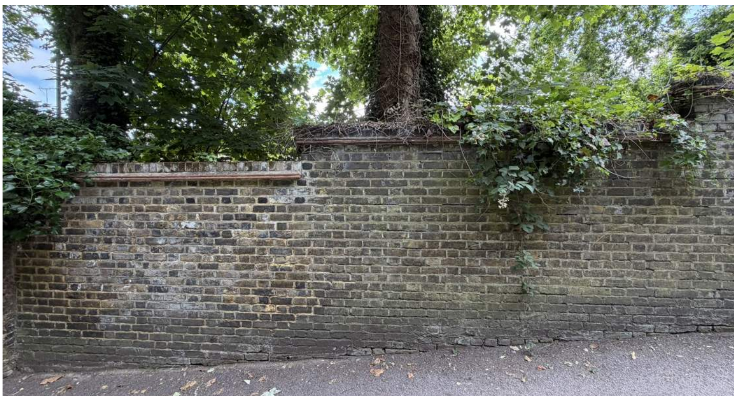
Photograph D - Showing steps in the boundary wall with a rotated header course at the top and a double tiled detailing and a simple predominantly yellow stock brick formation below. There is no grey/blue plinth stone within the wall at this location.
