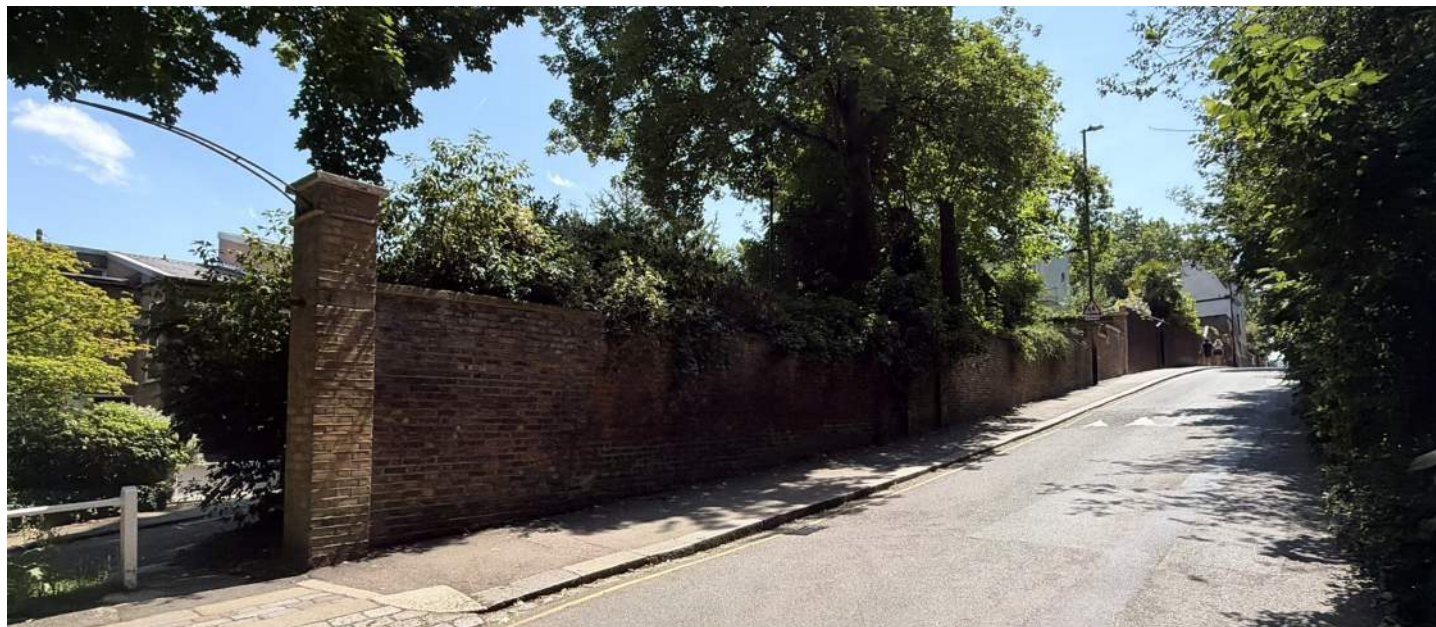
Photograph A - Showing rebuilt original entrance pillar to Southwood House in a predominantly yellow stock brick which is in contrast to the mixed red stock bricks from the wall adjacent. The entire wall can be seen sloping upwards along Southwood Lane.
