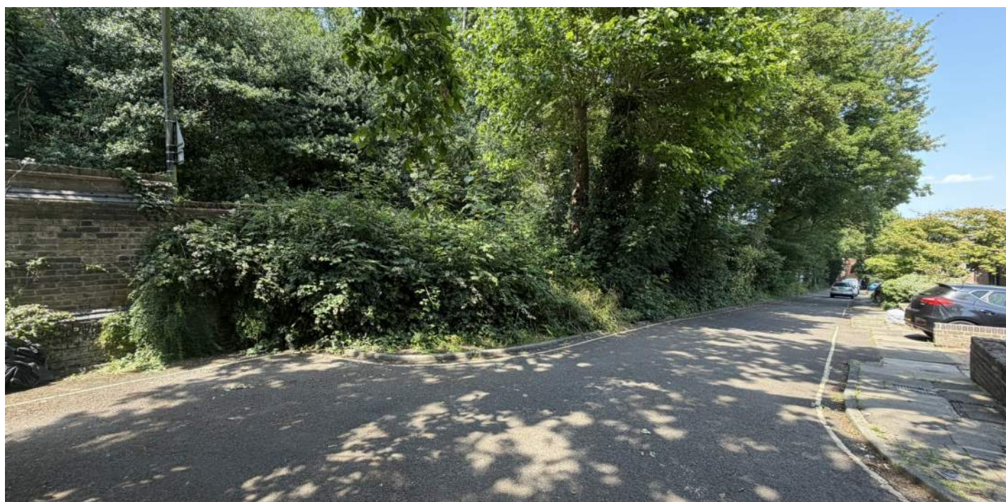
Photograph G - Looking along the length of the boundary wall towards the North. Dense evergreen planting hides the vast majority of the boundary wall from this side.
