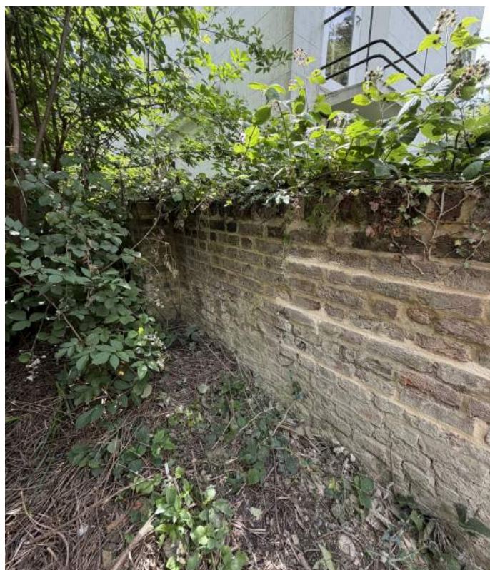
Photograph O - Shows a small portion of yellow stock bricks with a vertical header course, there are no coping or plinth stones along the length of this wall.
