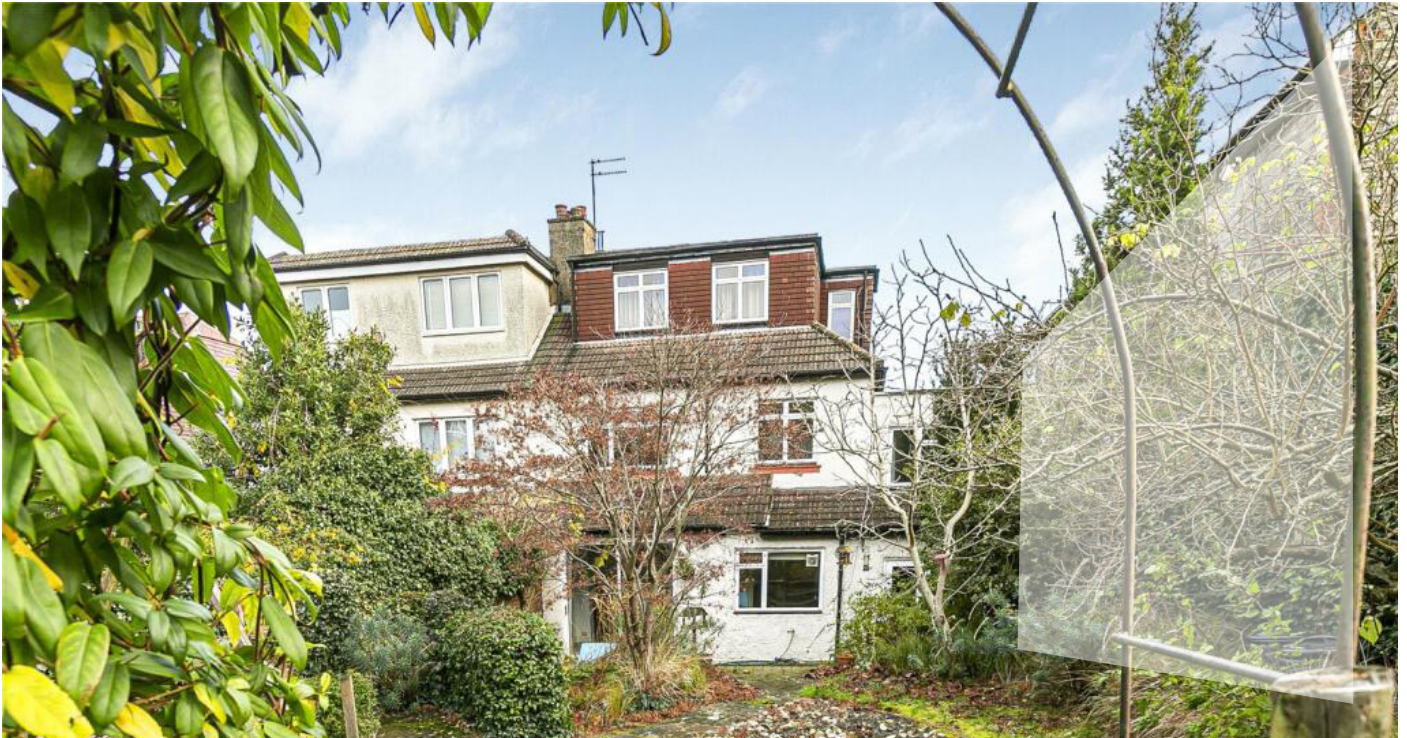
View of house from garden. Note: flank wall of No. 69 shown in white.
