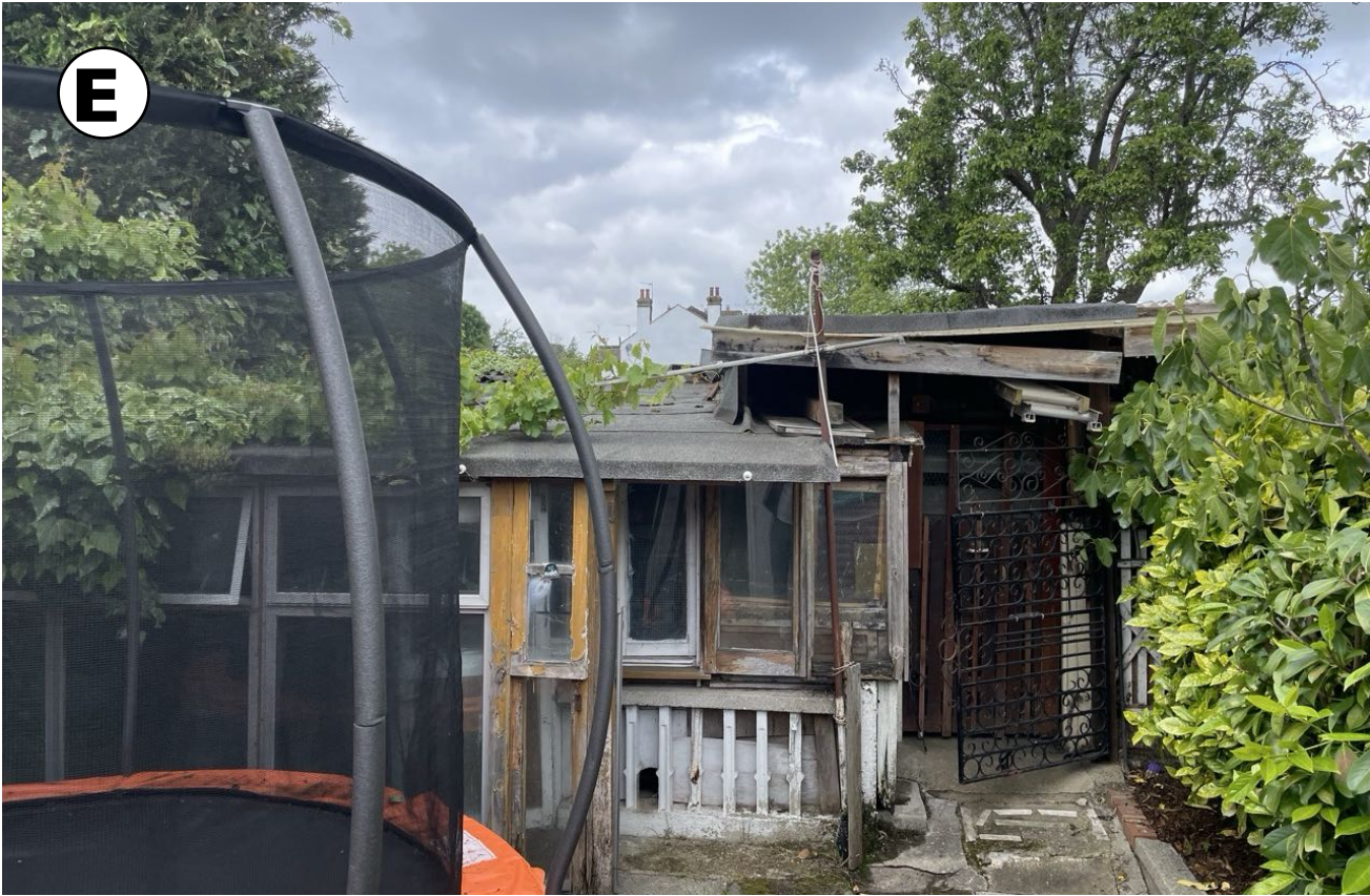
Photo from the garden looking west towards the garden elevations of the existing garden structures C and D
