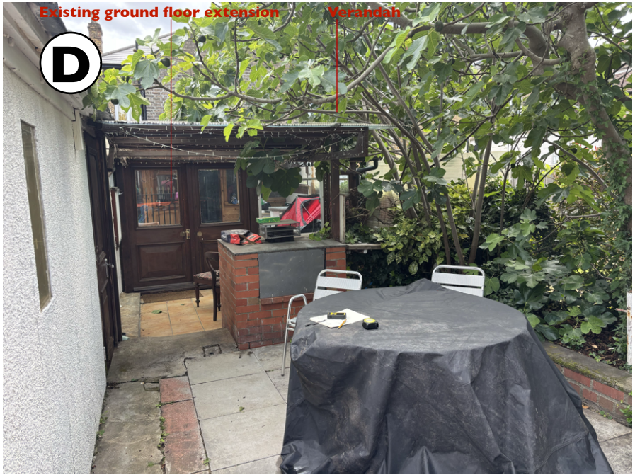
Photo from the verandah in front of the existing ground floor extension
