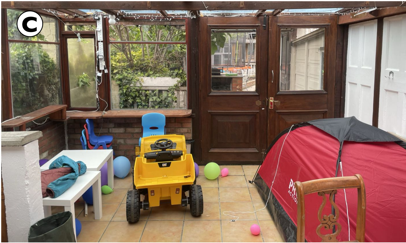
Photo from the house showing the internal view of the existing ground floor extension
