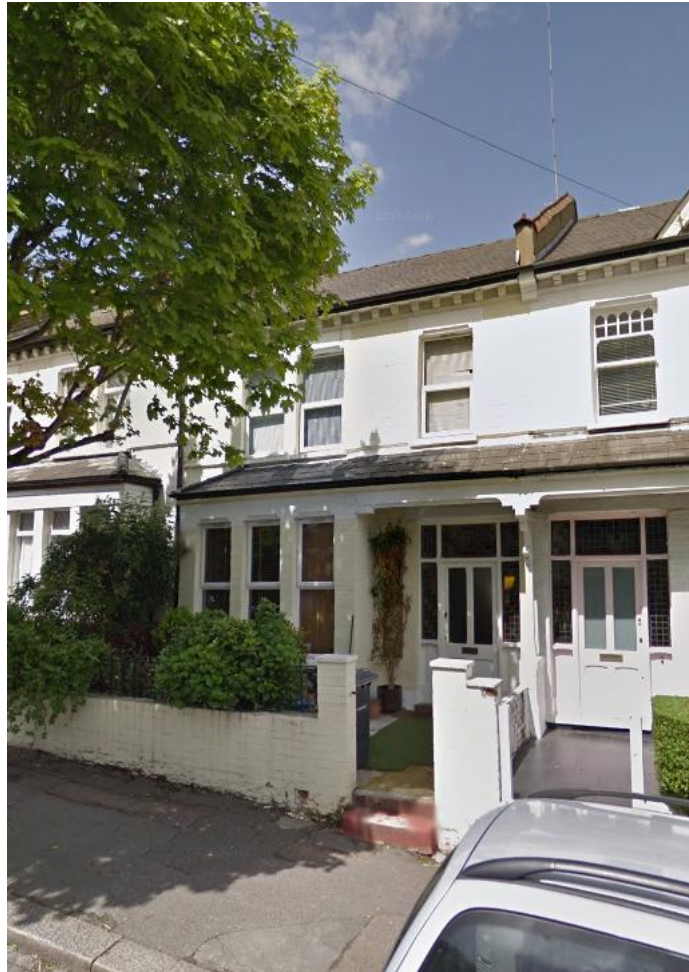
View of application site
