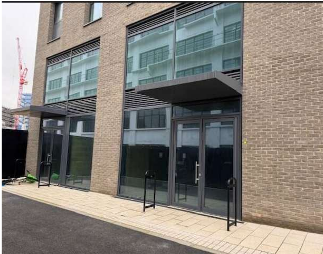
Finished Curtain Walling to Commercial Units for Block E2
