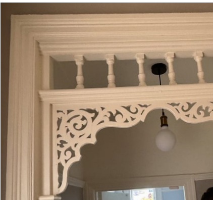
HISTORIC DETAILS Decorative internal panelling
