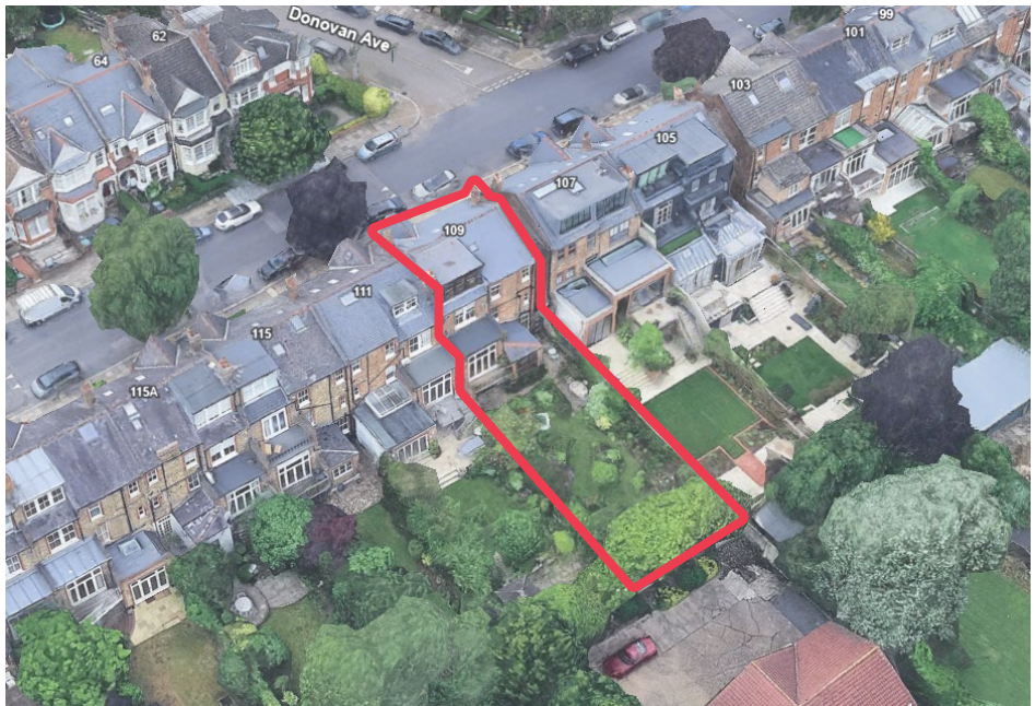
SITE AERIAL Aerial view showing 109 Rosebery Road (outlined in red) and the immediate neighbouring context
