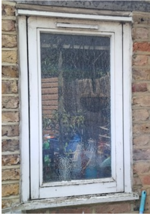
Rear Ground Floor Window
