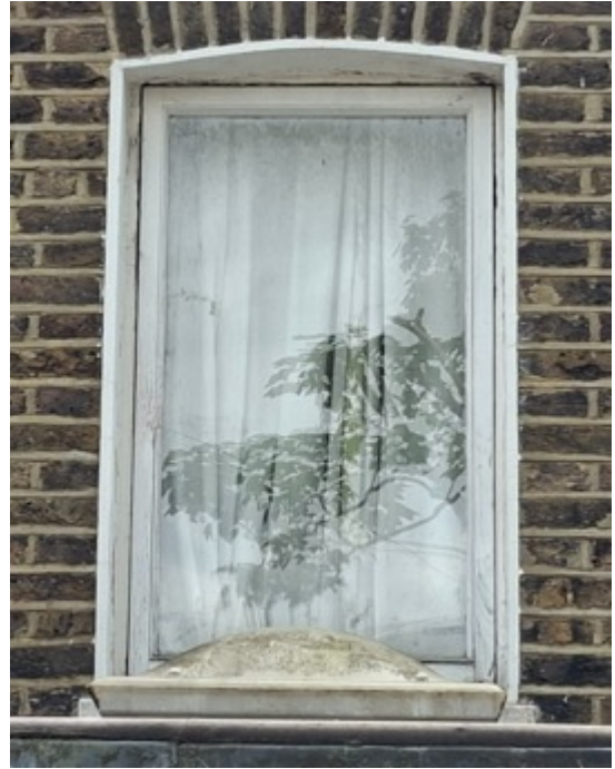
Rear First Floor Window
