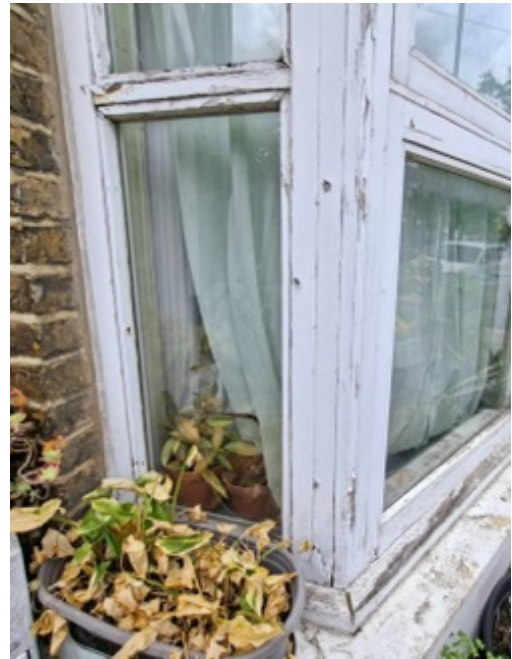
Front Ground Floor Bay Window (side view)
