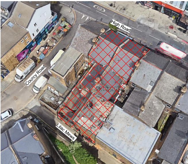
High Level North West Image
