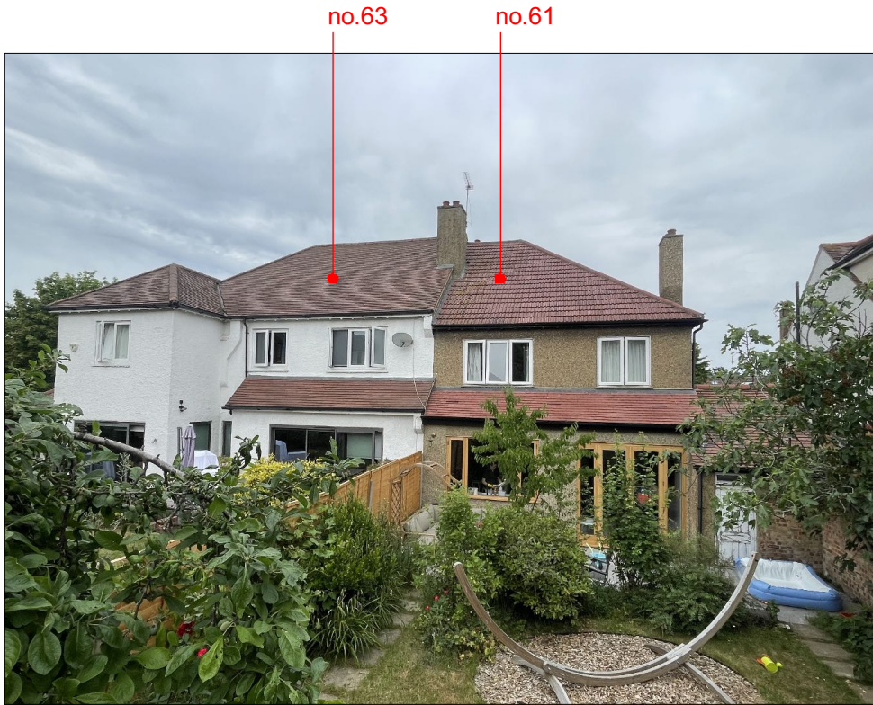
4. rear view of property and neighbouring properties
