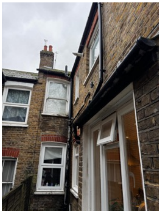
Rear & Rear Side Ground Floor Windows
