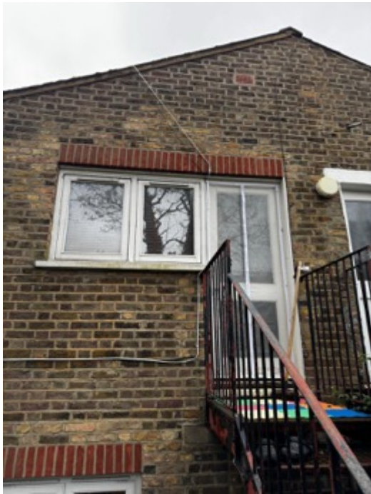
Rear End First Floor Exit Door
