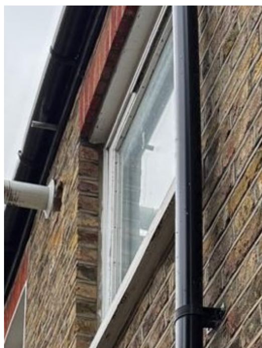
Rear Side First Floor Window
