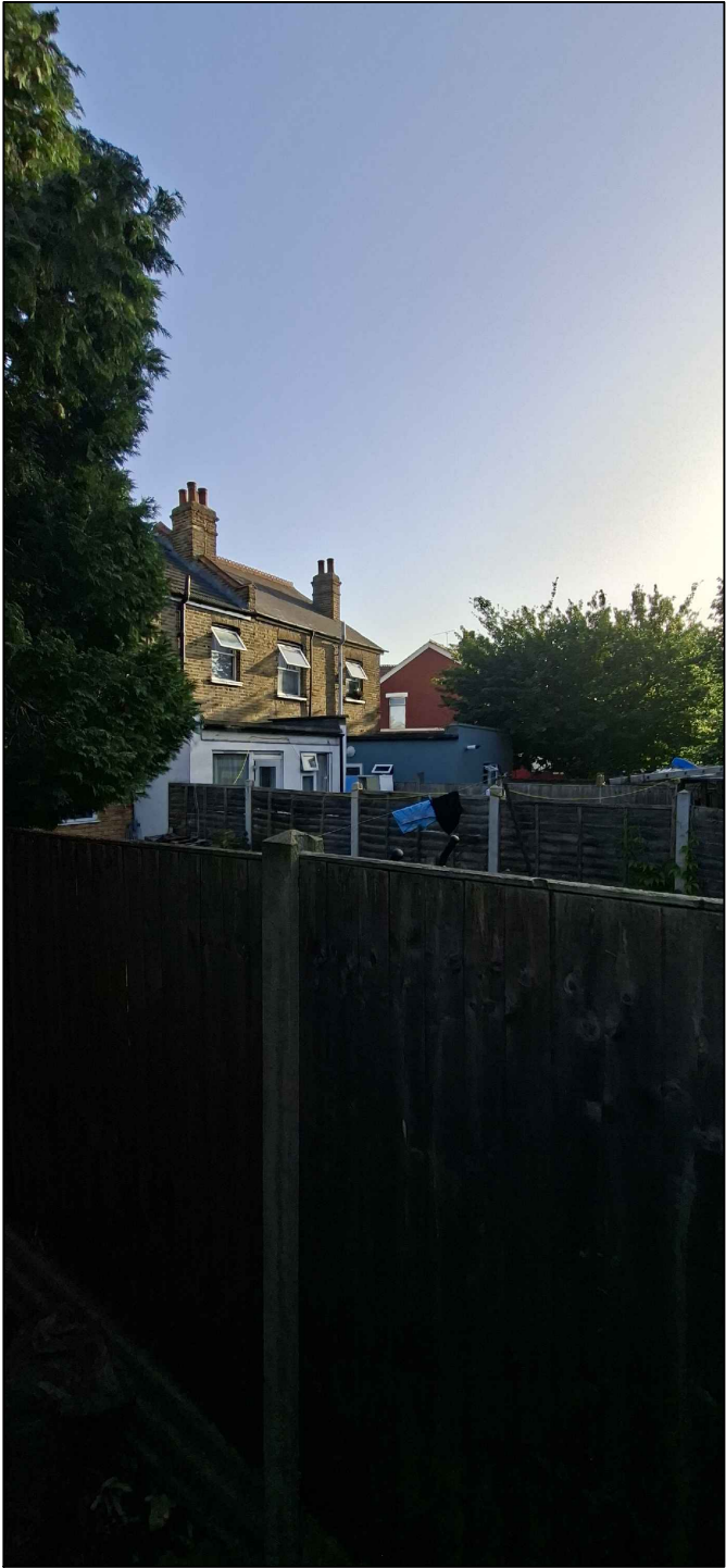
Rear elevation adjacent with No. 71
