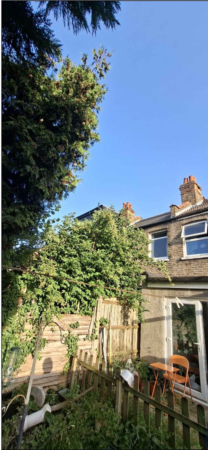
Rear elevation adjacent with No. 75
