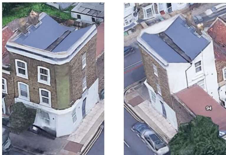
Google Earth images showing the loft conversion and roof design at 94 St Paul's Road
