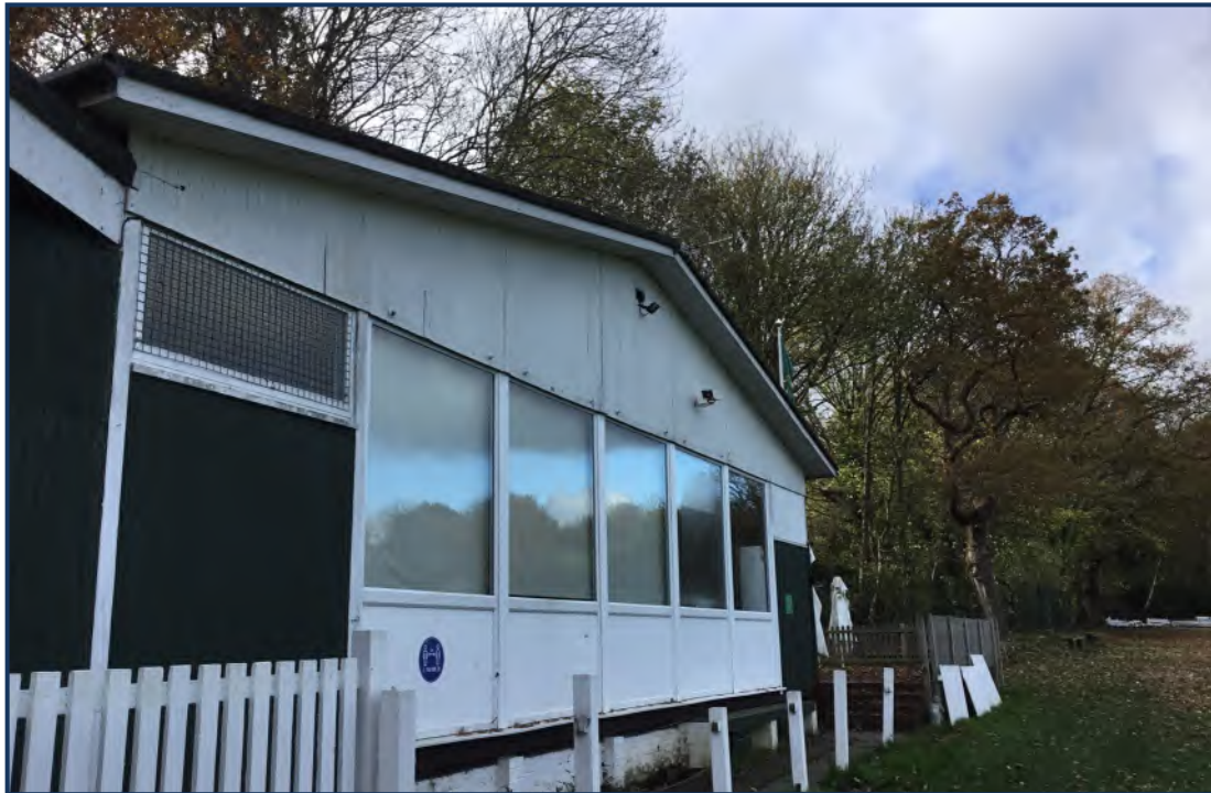
PHOTOGRAPH 1: Building B1 - Northern Elevation
