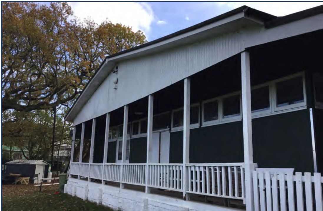
PHOTOGRAPH 4: Building B2 - Northern Elevation
