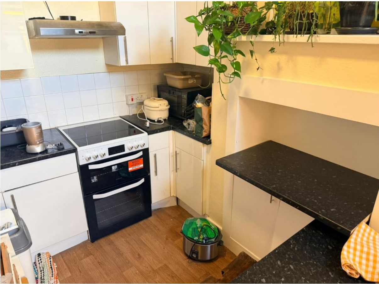
PH1 - New hob, oven, extractor, cabinets & worktop to the chimney in the kitchen
