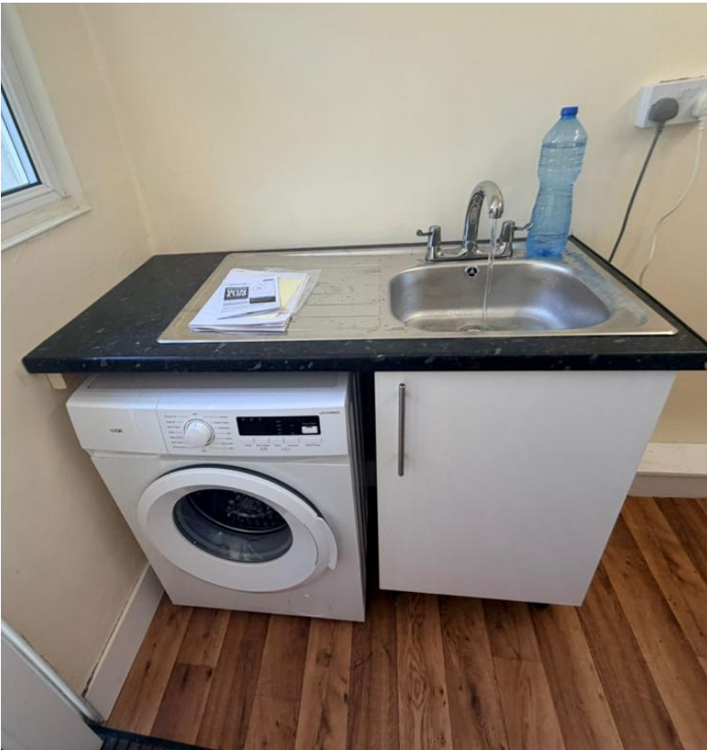
PH3 - New sink & cabinet in the utility
