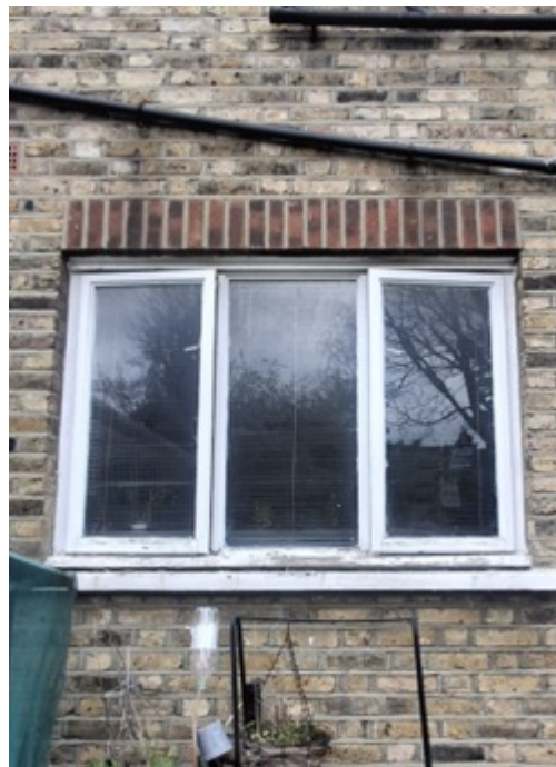
Rear Ground Floor Window
