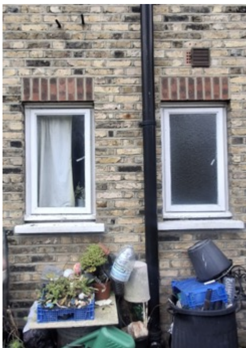
Rear Ground Floor Windows
