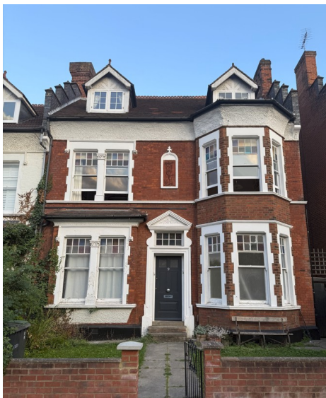
Image 2: Photo of existing front elevation
