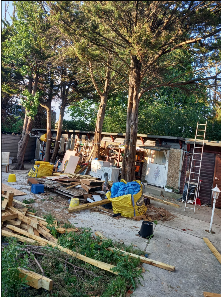
Picture 2. Shows the bottom of the garden with the existing tree and the outbuilding behind the trees. There is a an exiting concrete slab that was poured years ago.
