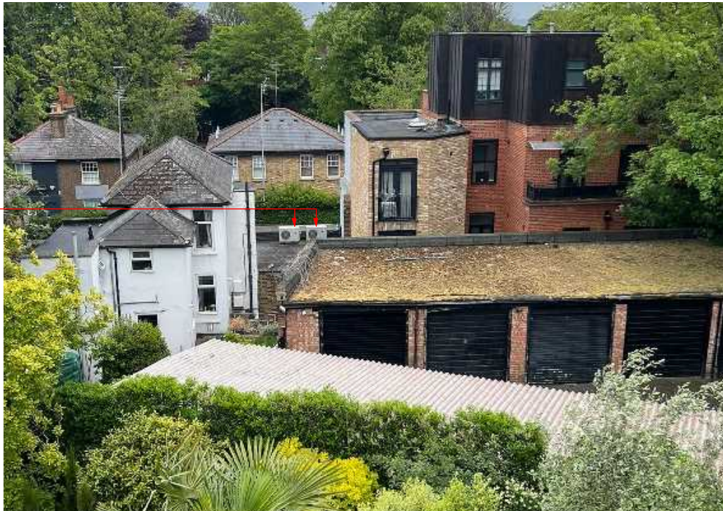
7. 636 Archway Road - view from the rear looking towards Archway Road
