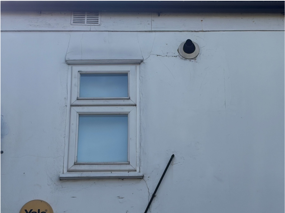
Photo 2: Existing kitchen window, left-hand first-floor window when viewed from outside. Taken 19 July 2026.
