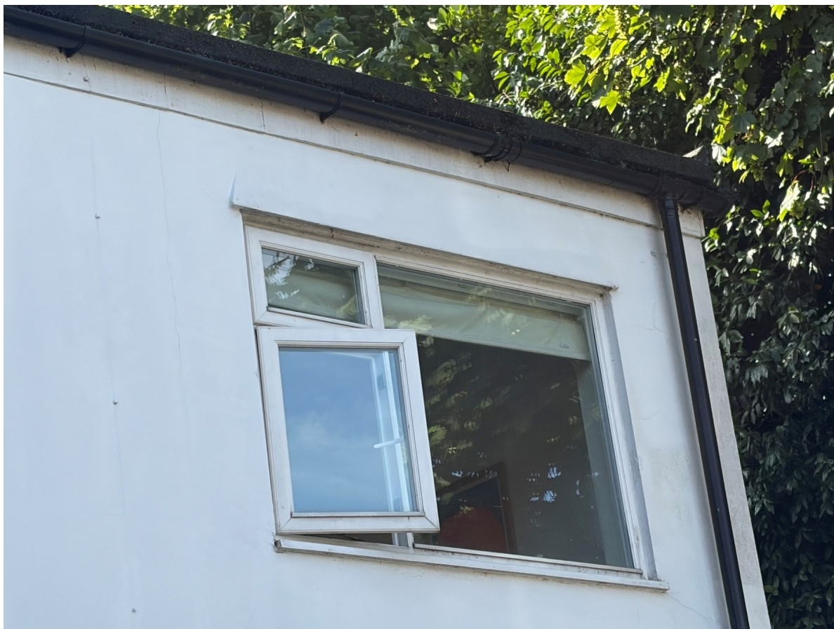
Photo 4: Existing bedroom window, right-hand first-floor window when viewed from outside. Taken 19 July 2026.
