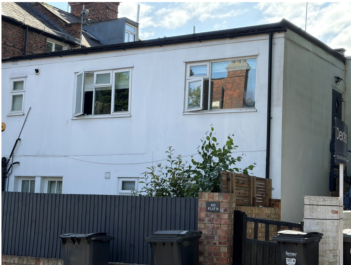
Photo 1: Context view of the Talbot Road-facing elevation showing the three first-floor 101 B Talbot Road windows, boundary fence, public pavement frontage and address signage. Taken 19 July 2026.
