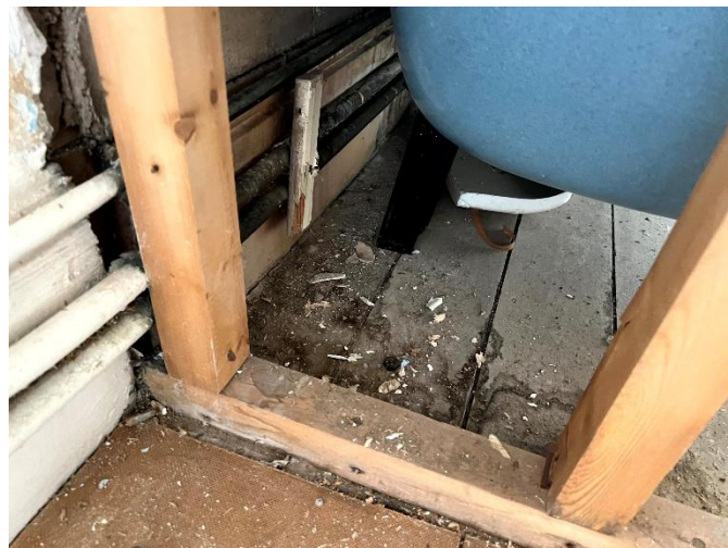
30 Exposed floor void and historic plumbing routes beneath bathroom. Illustrates extent of previous interventions to original floor structure.
