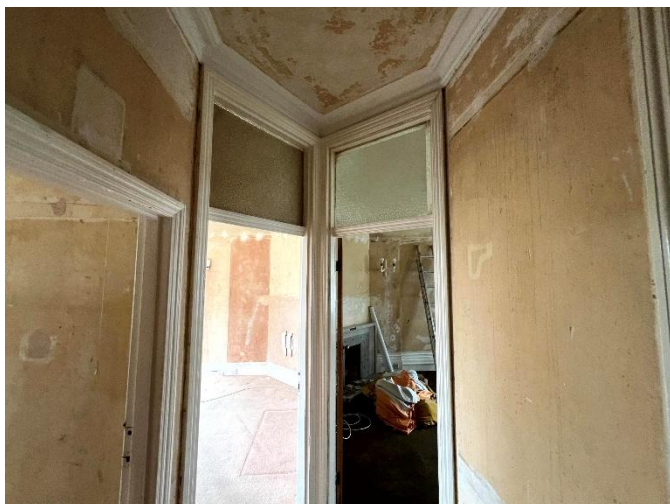
25 View through principal circulation route illustrating retained historic plan form and over-door glazing details characteristic of the Edwardian layout.
