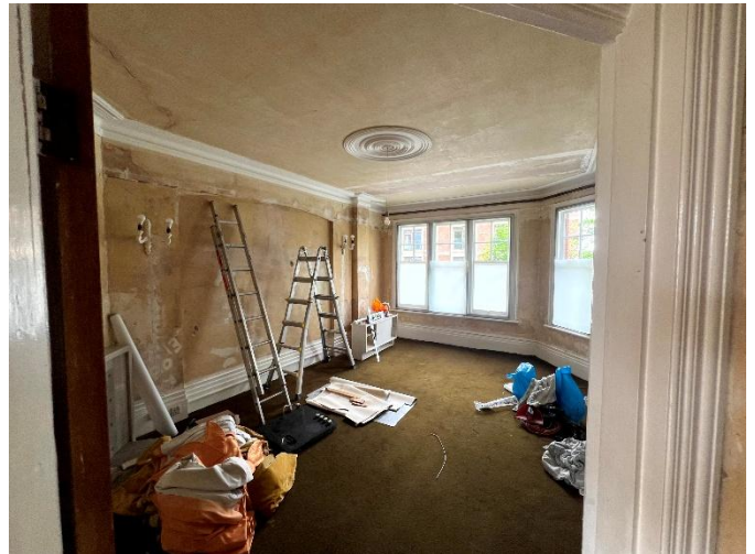
44 General view of principal reception room retaining original proportions, cornicing and window arrangement characteristic of the building's Edwardian design.
