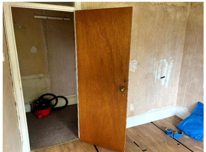
18 Secondary view of later replacement internal door and stripped wall finishes exposing underlying historic plaster construction.
