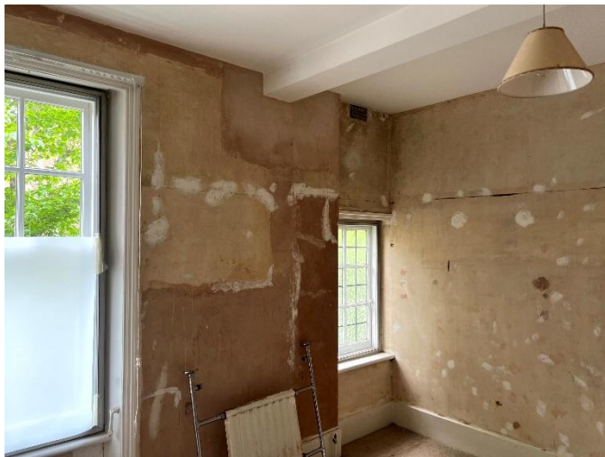
55 View of boxed bulkhead/downstand structure spanning across the room at high level. The formation is likely associated with a historic alteration involving either removal of an earlier partition wall and/or concealment of structural strengthening and service installations undertaken during a previous refurbishment phase. The bulkhead does not appear consistent with the original Edwardian ceiling arrangement and is considered a later intervention of limited heritage significance.
