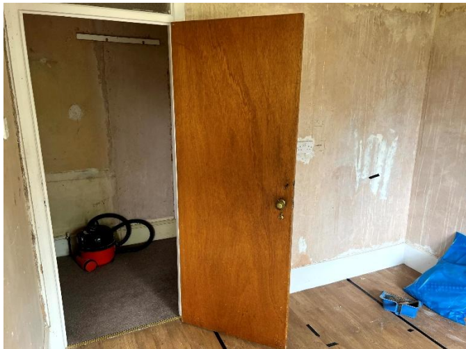
13 Internal doorway and surviving historic room proportions. Existing timber door appears to be a later replacement rather than original Edwardian joinery.
