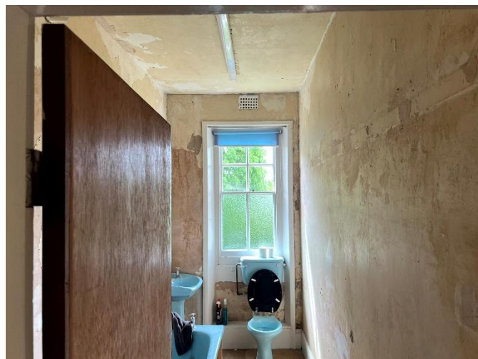
26 Bathroom arrangement showing original room proportions and retained historic window opening. Existing sanitaryware appears later twentieth century insertion.
