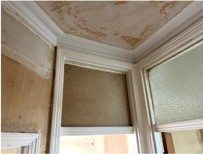
31 Original over-door obscured glazing panel with moulded timber surround. Important surviving historic feature proposed for retention.
