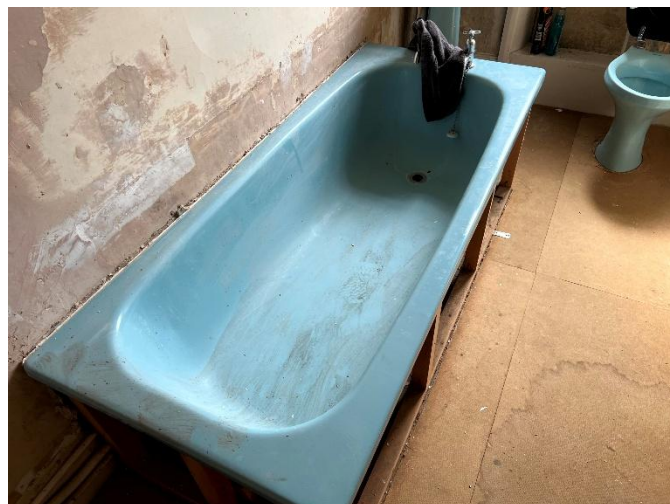
28 Existing bath installation of later date and limited heritage significance. Proposed replacement considered acceptable in principle.
