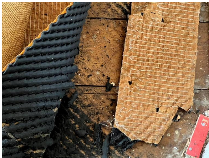
40 Close-up of historic floor finishes and adhesive residues associated with earlier coverings.
