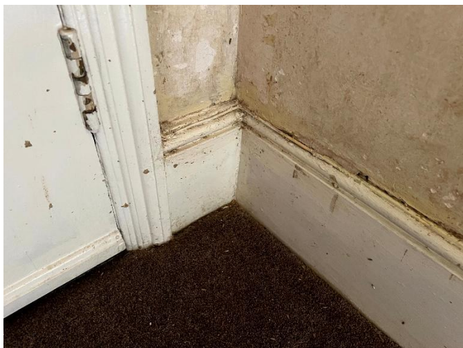
9 Original deep timber skirting and architrave detailing within hallway. Historic joinery largely retained although showing evidence of wear and previous decoration build-up.
