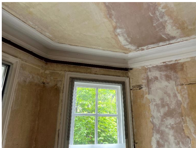
50 Original Bay window arrangement with moulded cornicing and retained Edwardian proportions. Important architectural feature of heritage significance.
