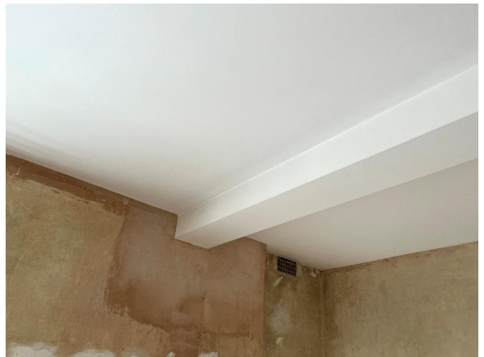
56 Secondary view of altered ceiling and wall arrangement showing boxed beam structure aligned with evidence of former wall junctions and historic alterations to the room layout. The lowered ceiling section and boxed enclosure are likely associated with historic remodelling works predating the current ownership and appear comparable to interventions approved within previous Listed Building Consent applications at The Gables, particularly where later twentieth century alterations and structural rationalisation had already materially affected the original fabric. Given the apparent age and established existence of the alteration, reinstatement of the original ceiling and partition arrangement would not typically be considered necessary as part of the current proposals, provided no further material alteration to the structure is proposed. The existing intervention is therefore considered part of the evolved historic fabric of the flat rather than a new unauthorised alteration arising from the current refurbishment works.
