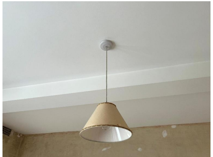
54 Replacement ceiling light fitting suspended from original ceiling position, which is not original. Proposed rewiring intends to retain existing lighting locations.
