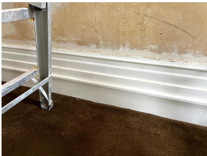
49 Original deep moulded skirting detail within principal room. Significant surviving historic joinery requiring protection during proposed works.
