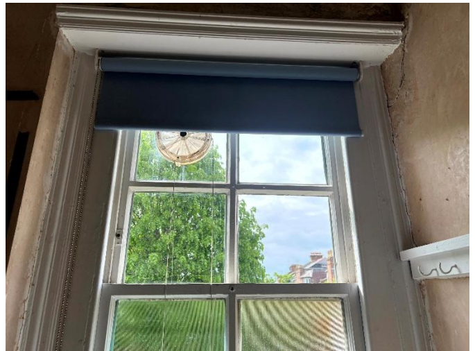
20 Original timber sash window and reveal detail within kitchen. Window contributes significantly to the character of the listed building and should be retained and repaired.
