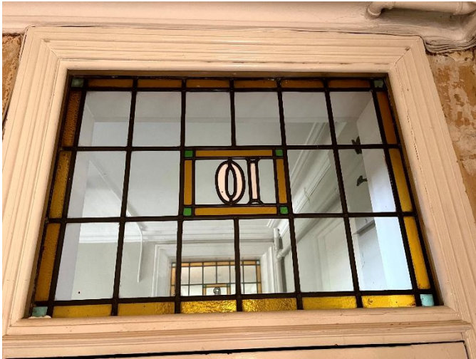
5 Original leaded and stained over-door light incorporating decorative glazing bars and flat number motif. Significant surviving historic feature proposed to be retained and revealed as part of refurbishment works.
