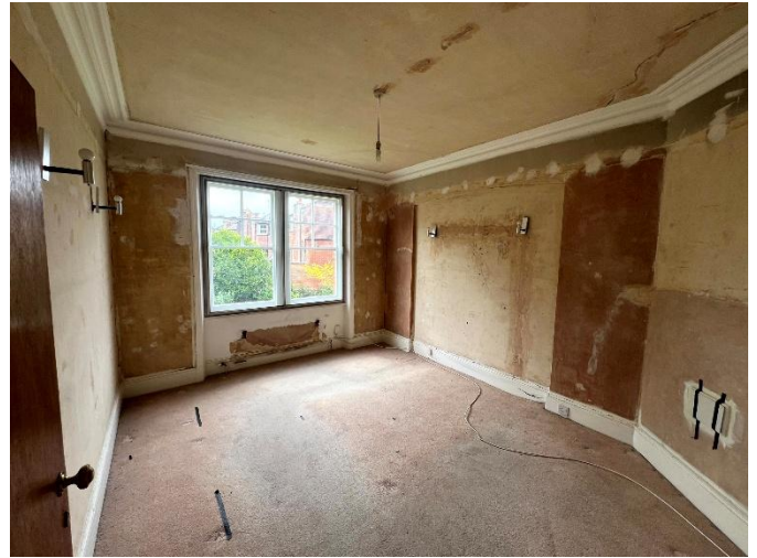
32 General view of bedroom 1 showing retained cornicing, window proportions and original spatial arrangement. Proposed works remain non-structural.
