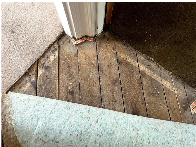
39 Exposed original timber floorboards adjacent to doorway threshold. Boards exhibit wear, splitting and previous disturbance associated with historic services.
