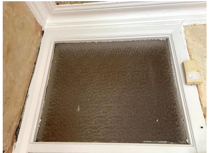
14 Original obscured glazed over-door panel with moulded timber surround. Historic feature contributing positively to internal character and proposed for retention.
