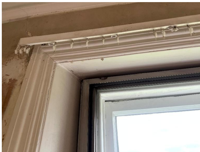
38 Original window reveal and moulded architrave detailing. Surviving historic joinery contributes positively to significance of the flat.
