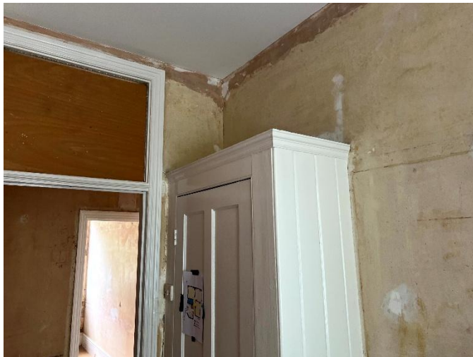
53 Surviving built-in storage joinery and upper over-panel detail. Cupboard arrangement likely historic and contributes positively to significance of interior.
