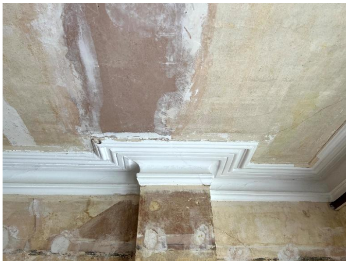
51 Decorative plaster cornice and ceiling junction detail. Original feature contributing positively to the architectural character of the flat.
