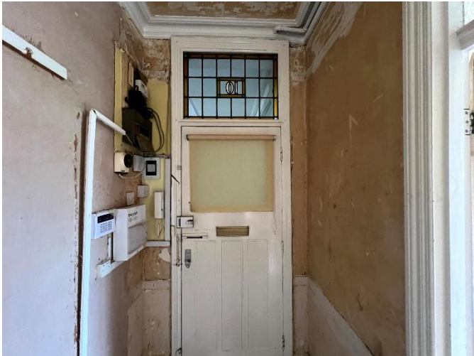
7 Hallway arrangement showing surviving original joinery, over-door glazing panels, cornicing and historic circulation layout. Proposed works comprise non-structural refurbishment and services upgrading only.
