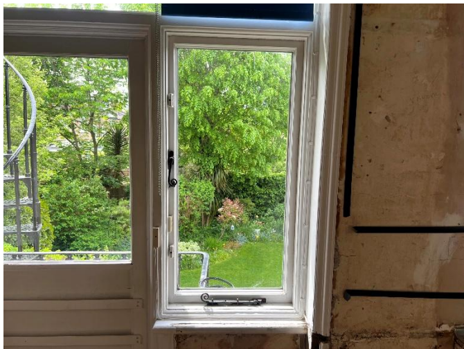
21 Original timber casement window arrangement with surviving historic proportions and glazing pattern. Repair-led approach recommended.
