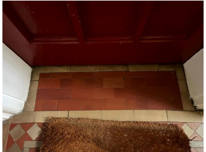
6 Original quarry tiled threshold and entrance flooring detail. Surviving historic floor finish of heritage significance requiring protection and retention during proposed works.
