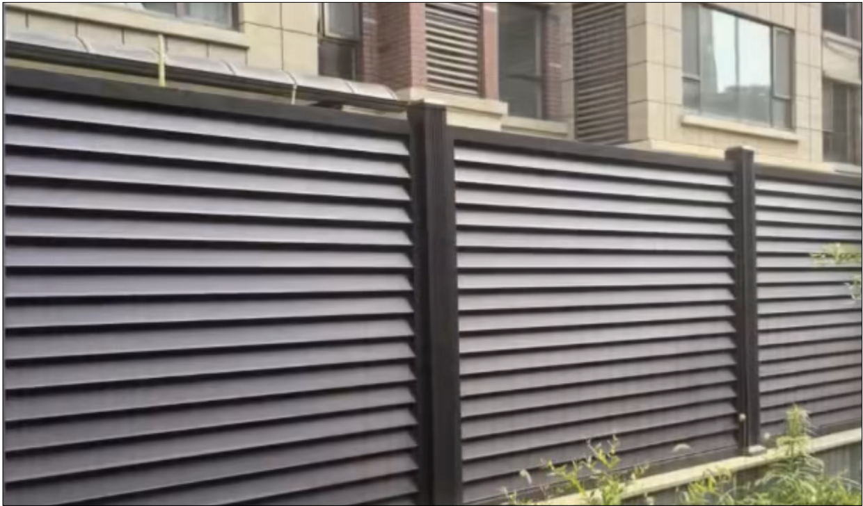
8. example of a horizontal slatted metal screen
