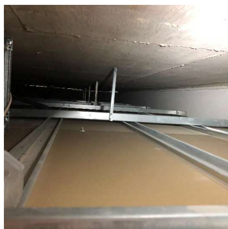
Left: views below the roof slab: in the service void
