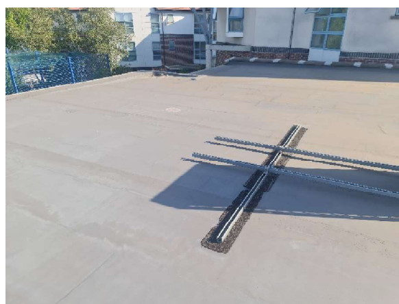
Above: views on the roof
