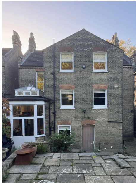
SITE PHOTOGRAPHY Rear Elevation of property
