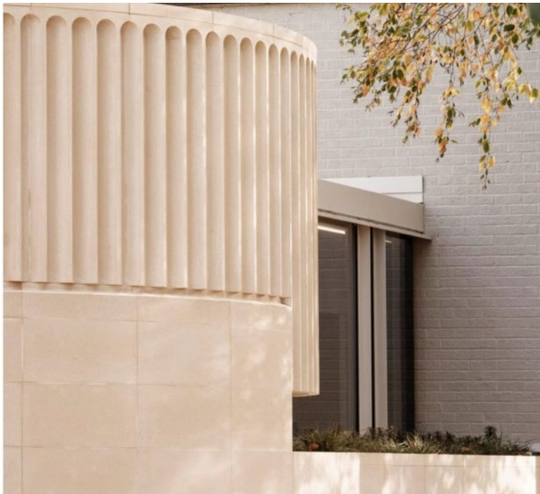
PROFILED STONE DETAILING A Light stone texture, such as portland stone, can produced a gentle rhythm and relief to the facade.
