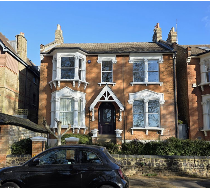
SITE PHOTOGRAPHY Front elevation of property
