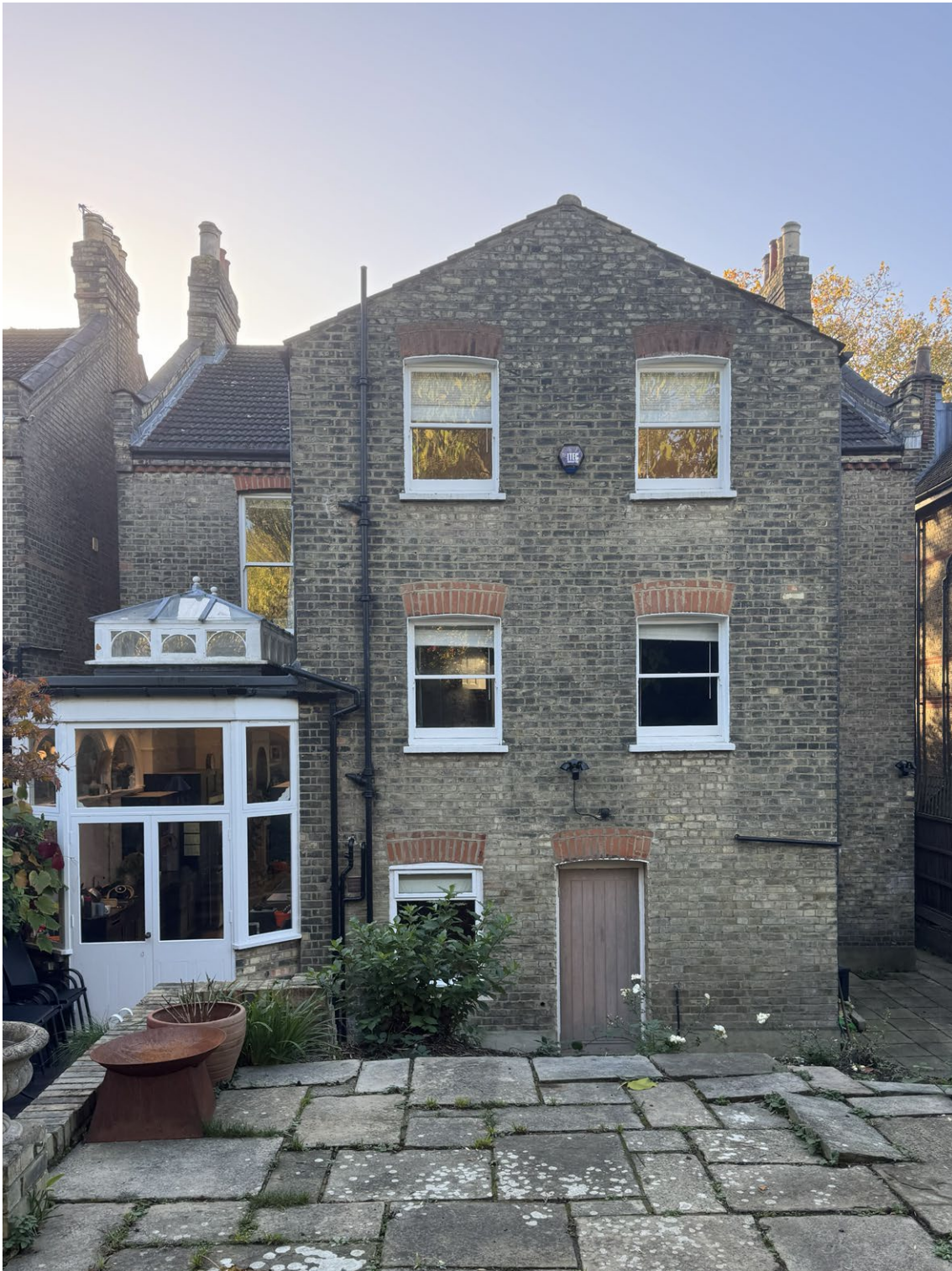
SITE PHOTOGRAPHY Rear Elevation of property
