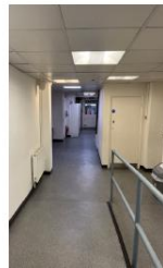
Fig. 5 (left) View of the pinchpoint in the corridor
