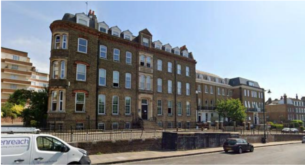
Figure 2: The 'Original' School Building comprising Channing House to left, with Slingley & Westview, along with Haigh House to right
