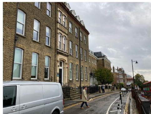
Fig. 2 The front elevation of Channing House with Slingley, Westview and Haigh House beyond
