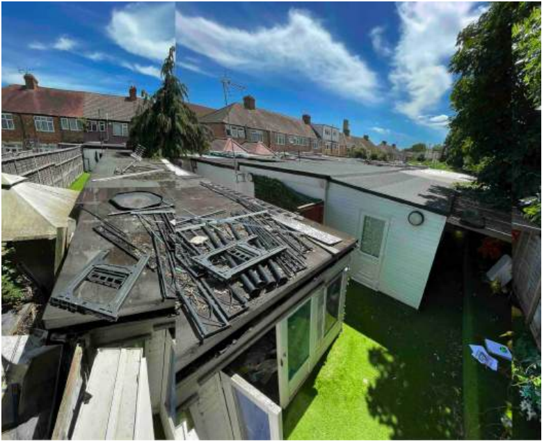
C VIEW LOOKING WITHIN THE SITE (BEHIND NUMBER 51) TOWARDS THE REAR OF 53, 51 + 49
