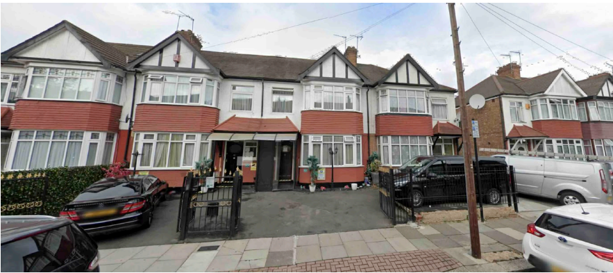
View looking at the front of 45 - 51 Pembury Road.
