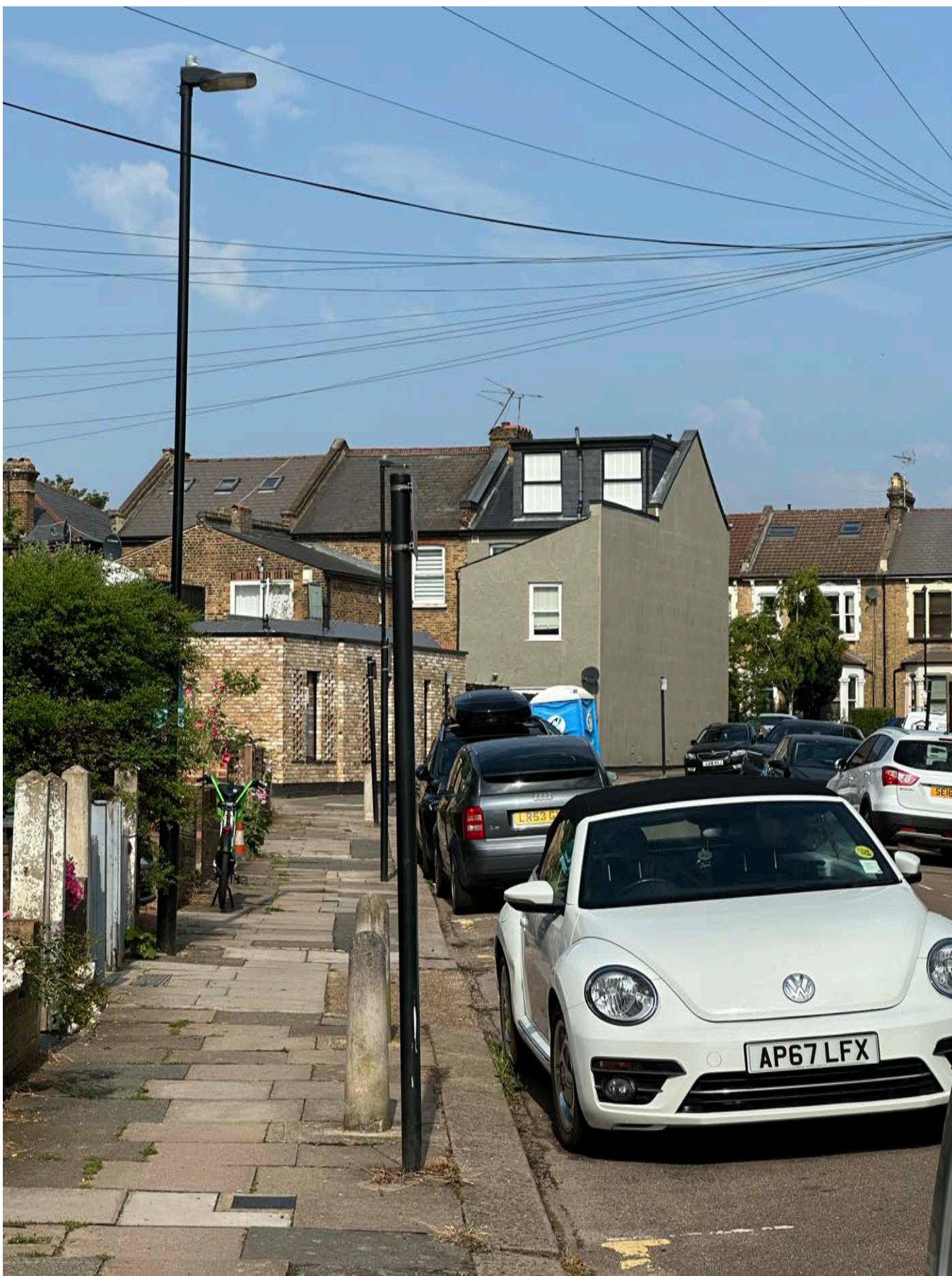
Photograph looking west from Thorold Road towards the dormer extension development at 44 Whittington Road
