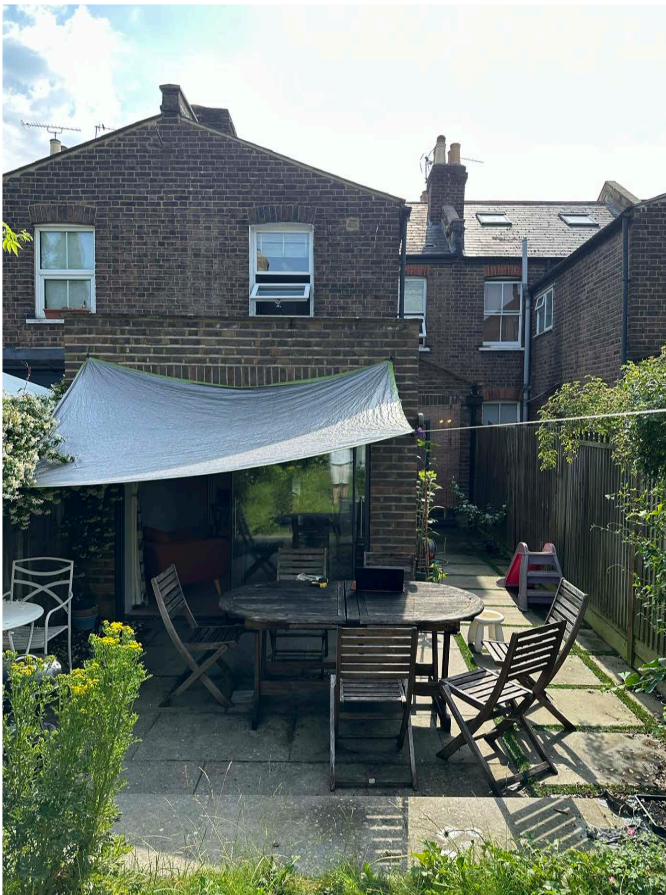
Photograph showing rear elevation of 21 Marlborough Road
