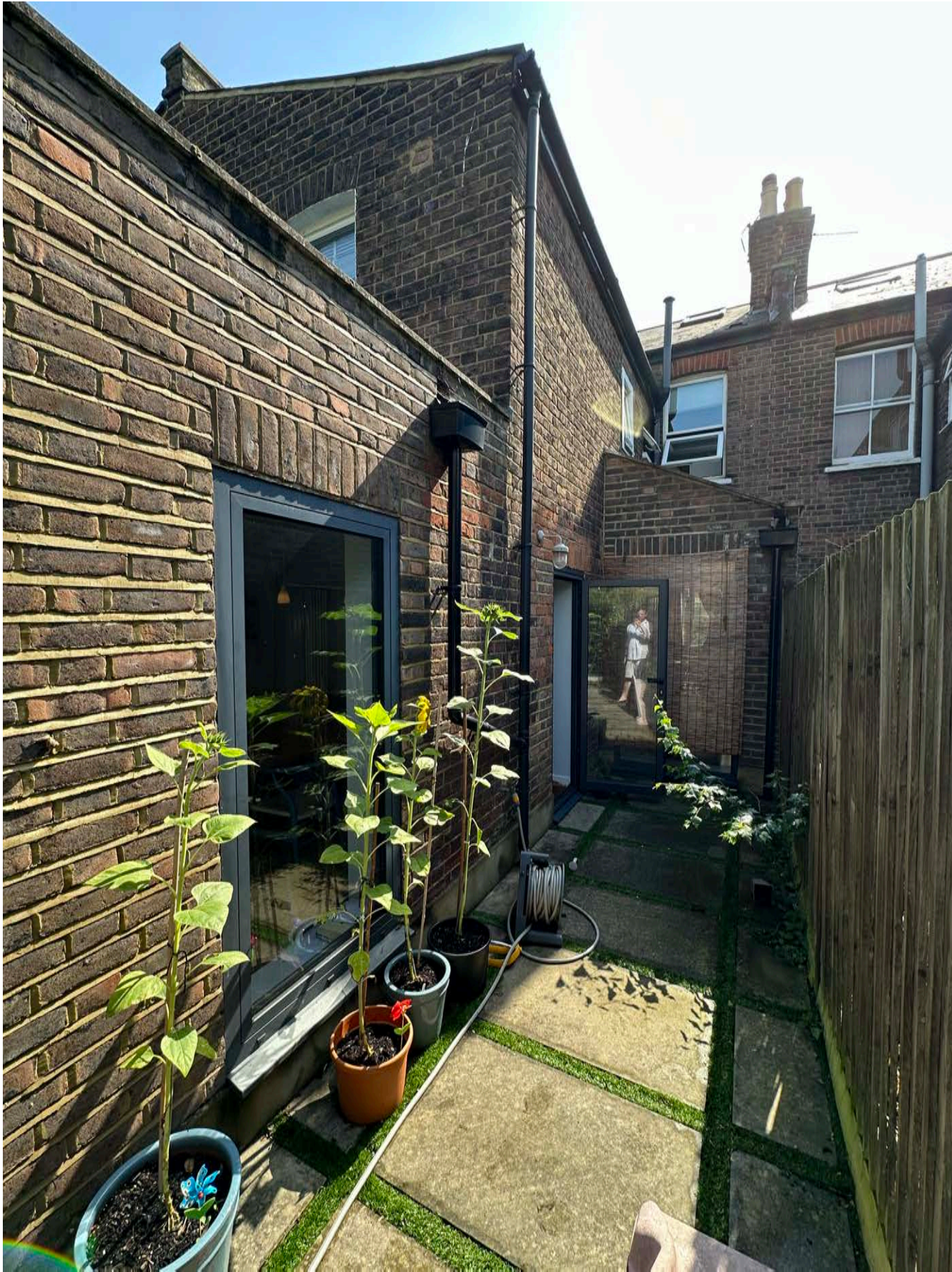
Photograph showing existing ground floor side and rear extensions at 21 Marlborough Road
