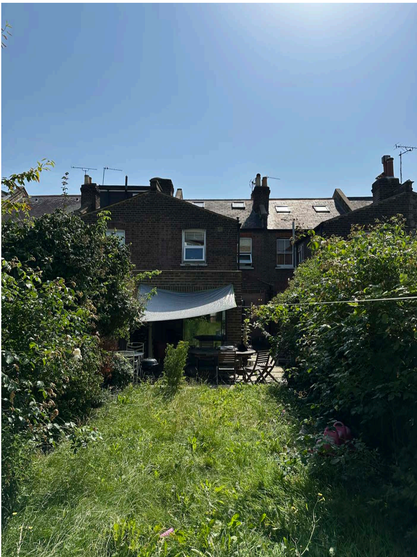
Photograph showing rear elevation of 21 Marlborough Road, seen from the bottom of the garden.
