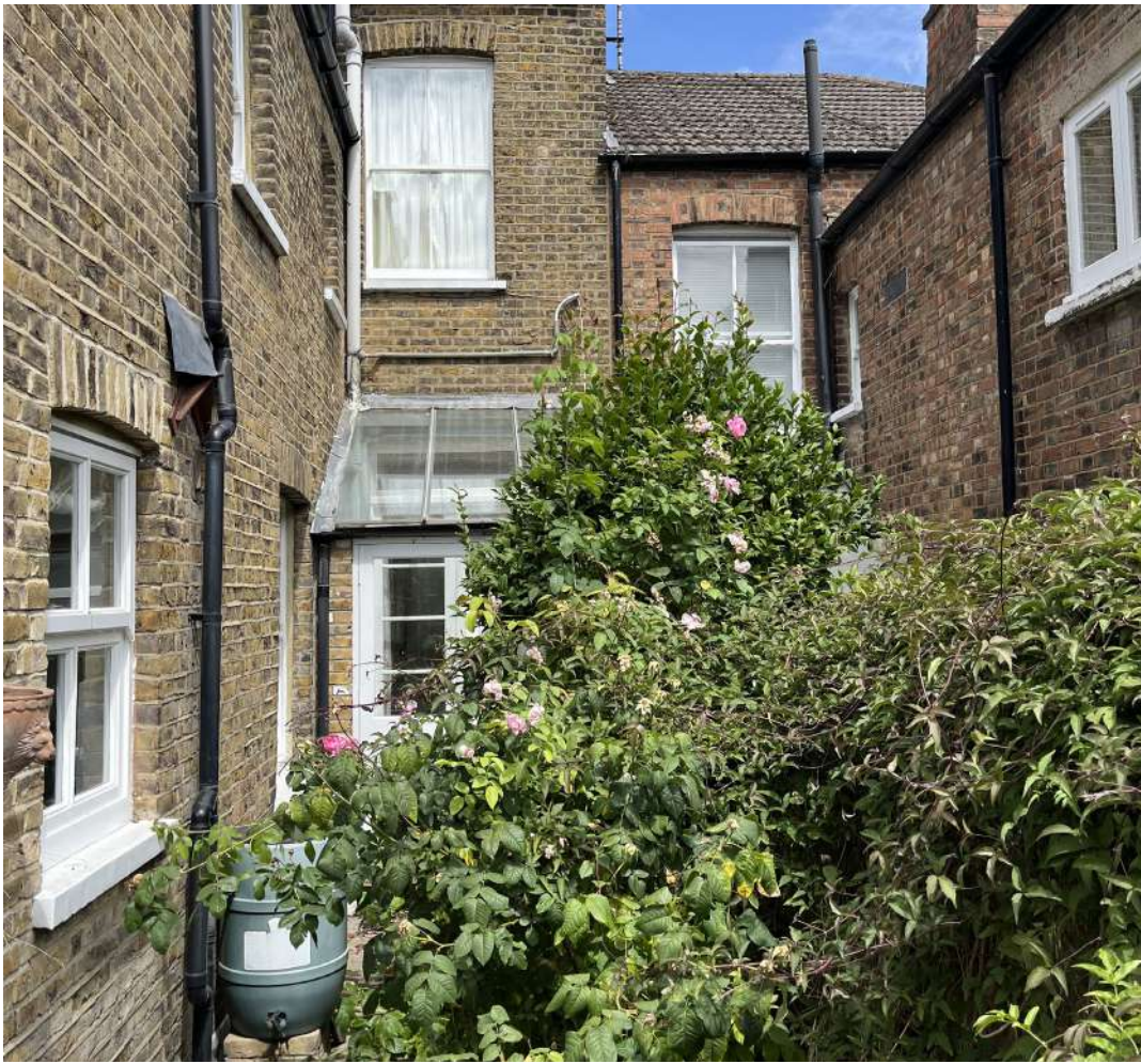
View of infill extension (date: 19/07/2026)
