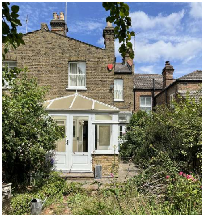
Views of front and rear of property (date: 19/07/2026).
