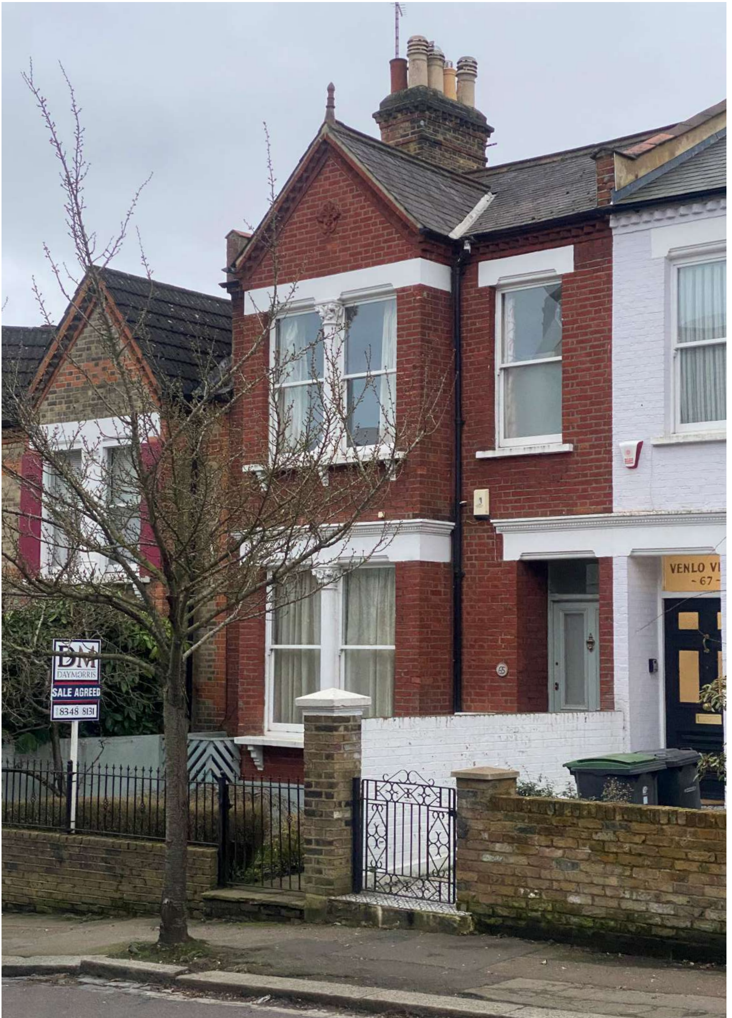
House Frontage (date: Feb 2026)
