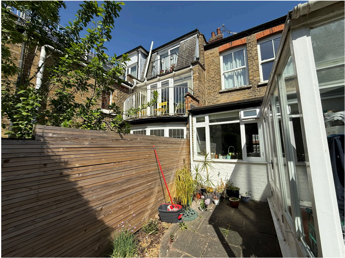
View of the rear / side boundary.
