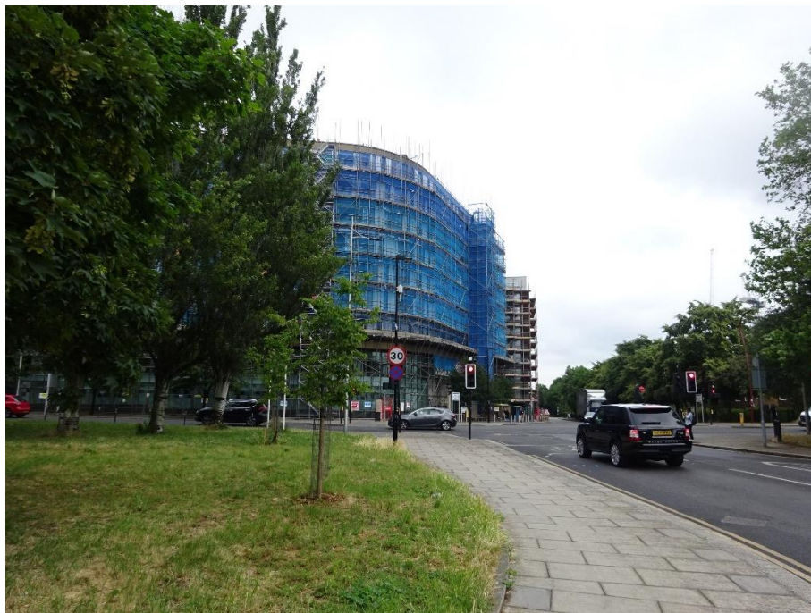
Photo 4: View of the site looking north.
